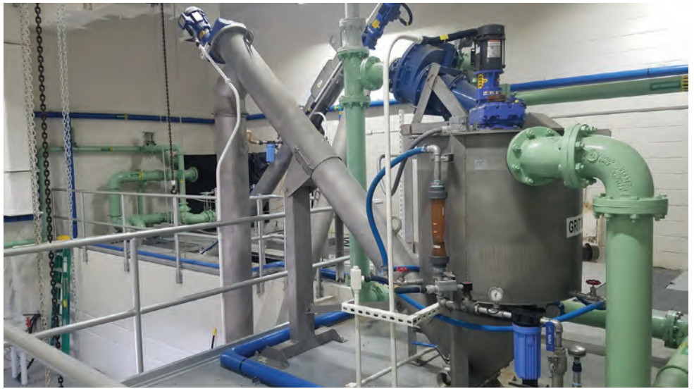
The Raptor Grit Washer (Lakeside Equipment) is designed to effectively provide grit classification and washing from any grit removal system.
