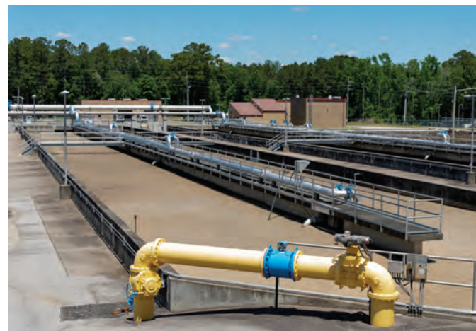
The Rockfish Creek Water Reclamation Facility.
