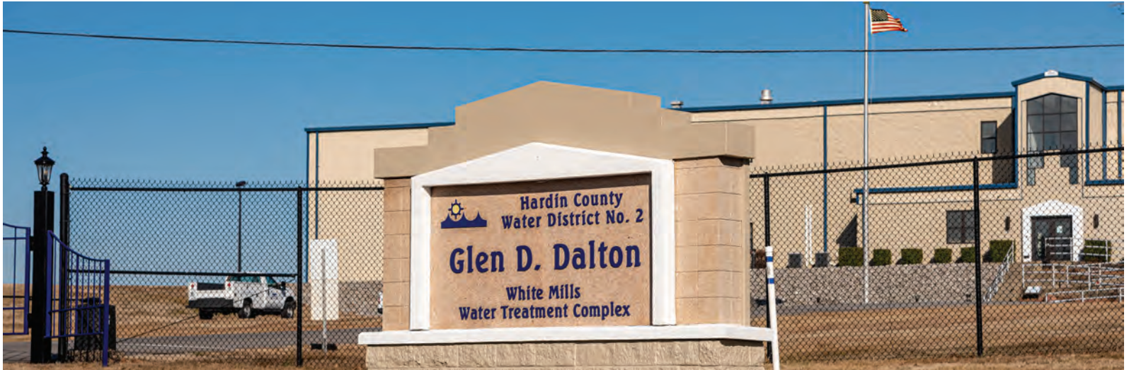
The White Mills Water Treatment Complex in Glendale, Kentucky.
