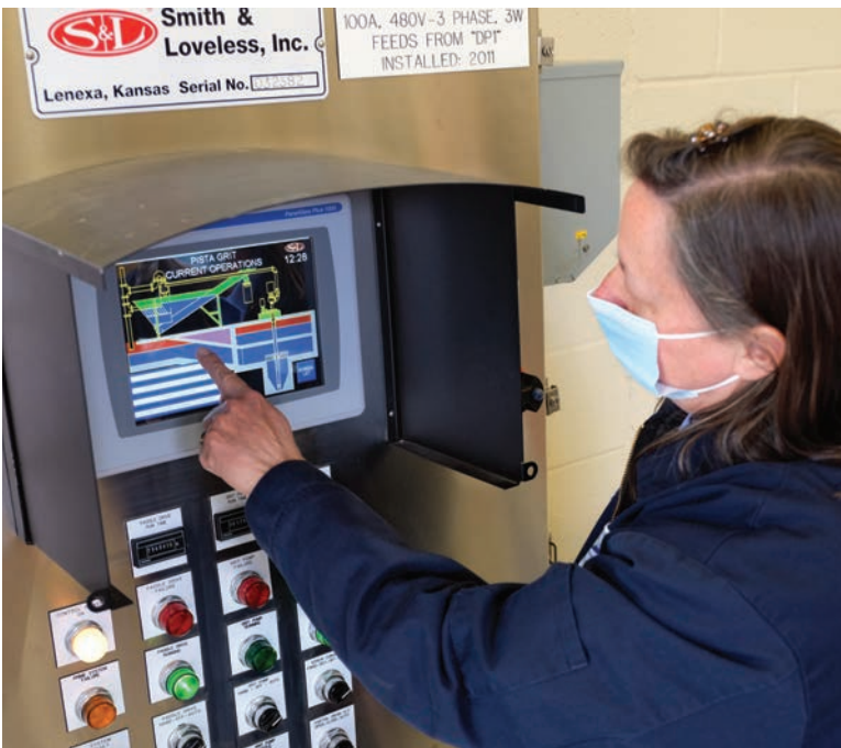
Sabine Wagner adjusts controls on the grit removal system (Smith & Loveless).
