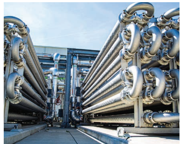
Heat exchangers recycle heat and help cool down the biosolids before they go to the digesters.
