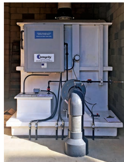
The I-BOx 6000 odor-control system (shown here at the Bluebird Lift Station) has provided reliable odor control for the City of Laguna Beach.
