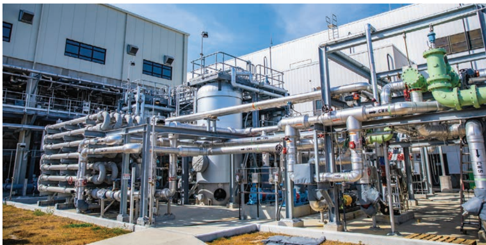
Some of the infrastructure for the thermal hydrolysis process at the Atlantic Treatment Plant.
