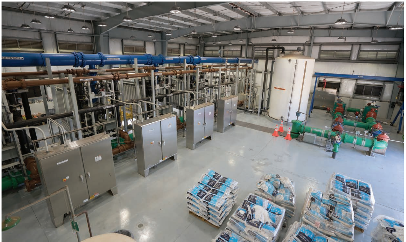
At the left are four continuous microfiltration units (Evoqua Water Technologies) in the Iao plant. Each can produce up to 1.50 mgd. The cabinets house the SCADA system servers and controls, developed and installed by Trimax.
