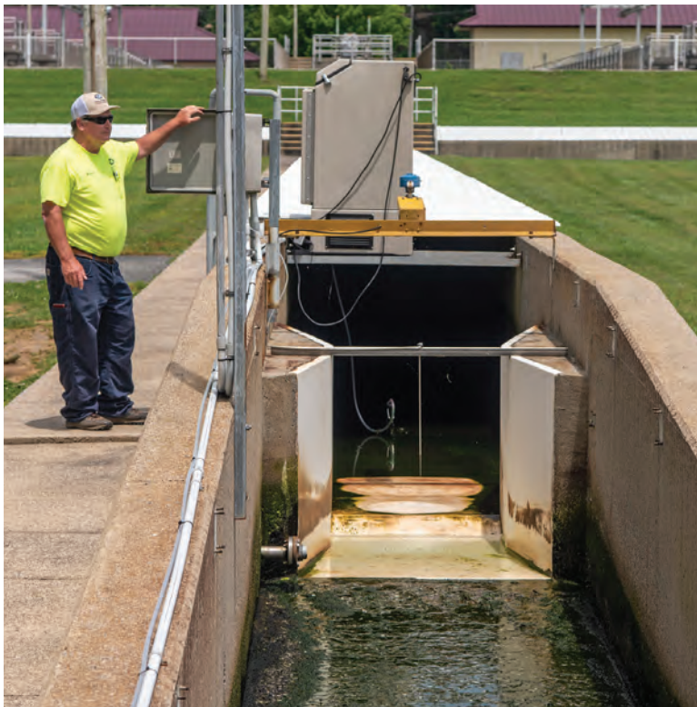
Plant supervisor Jeff Totherow refers to Bryan Gordon (shown checking the peracetic acid drip disinfection system from PeroxyChem), as the facility’s MacGyver for his inventiveness and problem-solving.
