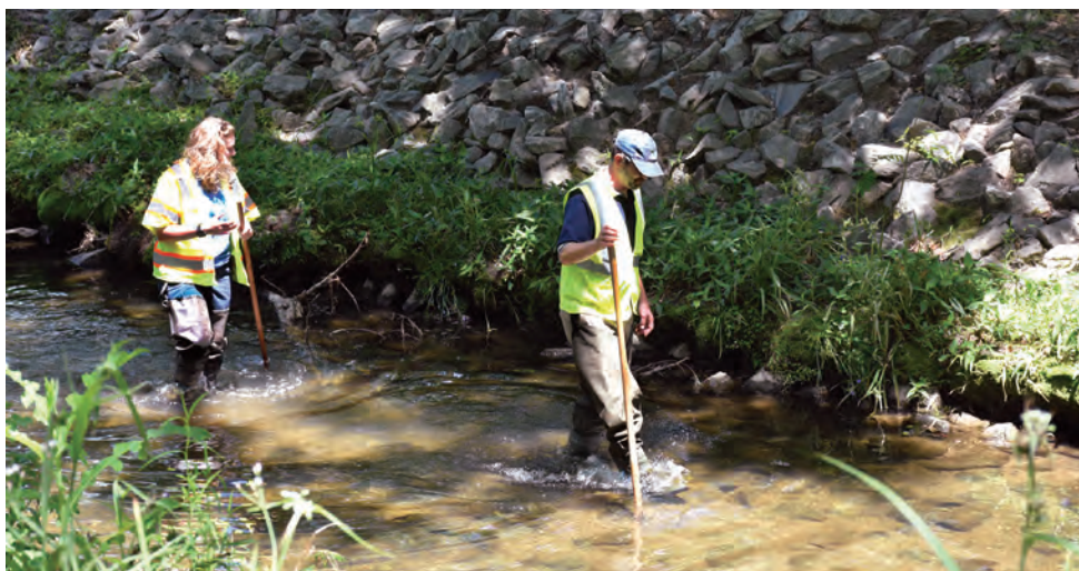
Columbus Water Works team members regularly wade upstream in creeks looking for problems such as cracked sewer pipes or erosion that has left pipes unsupported.
