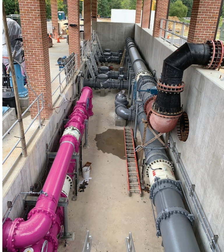
The room hosting UV disinfection equipment is shown within a building under construction. The finished project is to include five UV channels.
