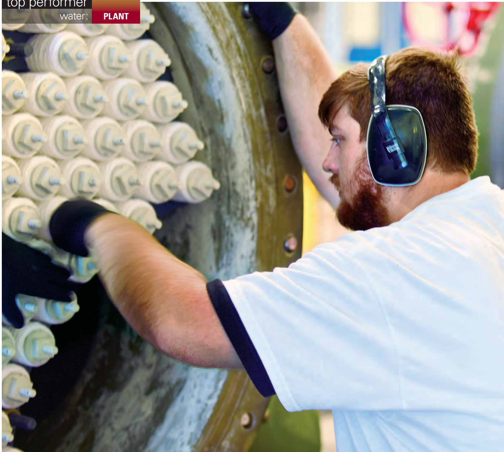
Operator trainee James Schaff replaces filter cartridges in the treatment plant's reverse osmosis system.
