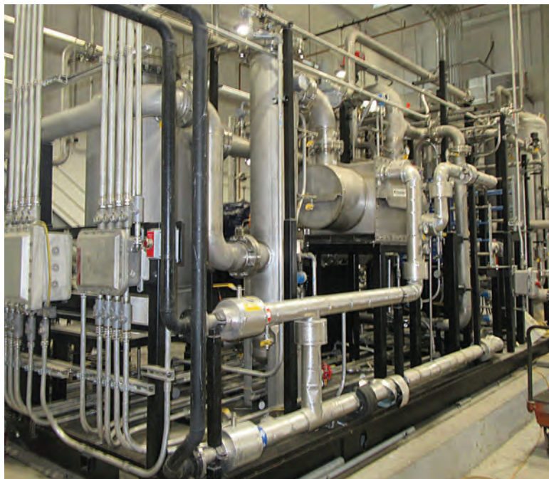
Unison Solutions gas carbon dioxide cleaning equipment was installed for the conversion from combined heat and power to producing pipeline-quality renewable natural gas for transportation fuel.
