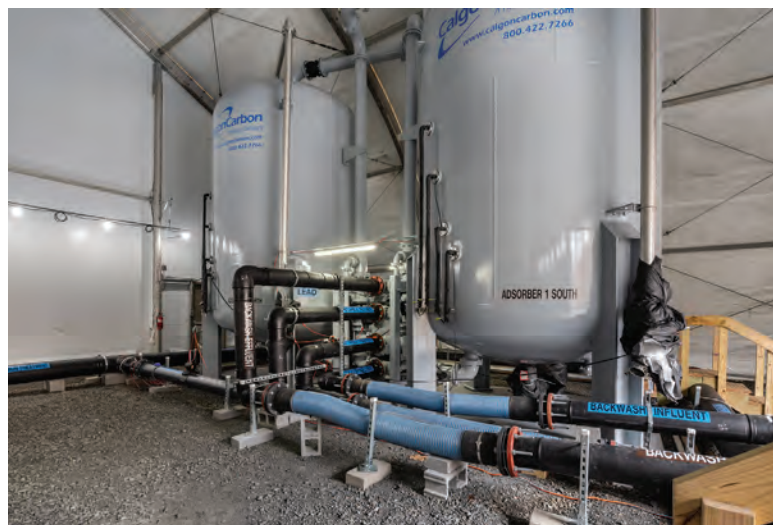
This granular activated carbon vessel pair is one of three at the Butterhill Water Filtration Plant in New York. Raw water flows top to bottom through the lead vessel and then through the lag vessel.
