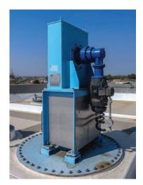
The Ovivo LM mixer on top of a digester at the Caldwell facility.
