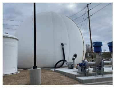
This "bubble" tank stores biogas at the plant.
