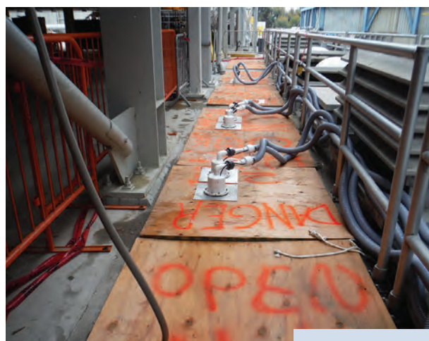
The covered influent channel with nozzles placed above.
