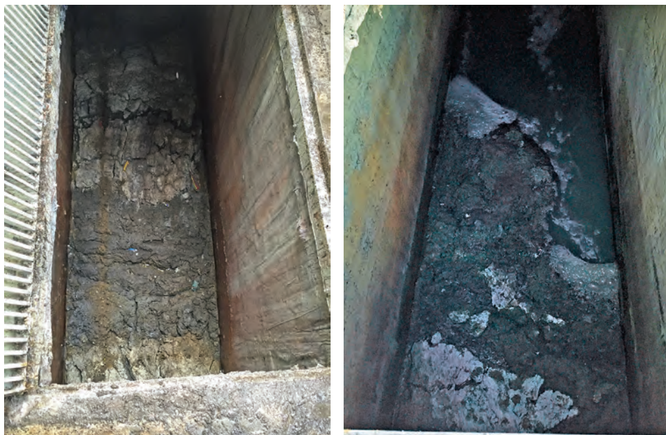
The FOG blanket was about 14 inches thick before trial started (left photo). Three weeks after the trial started, influent water could be seen.
