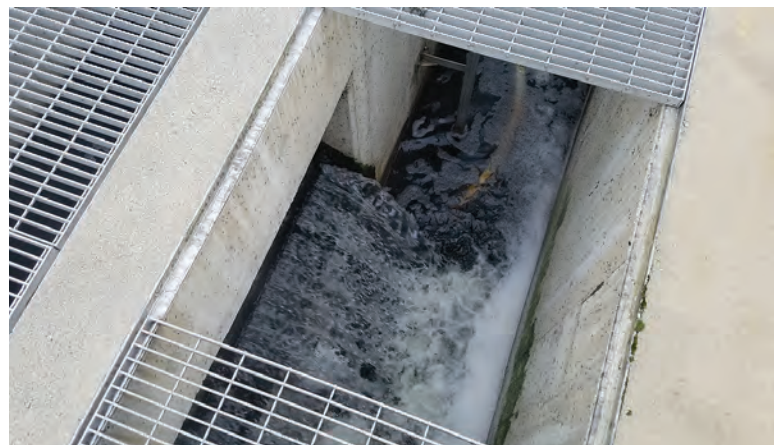
Overflow from the filtration building provides enough agitation to mix chlorine in the disinfection tank.
