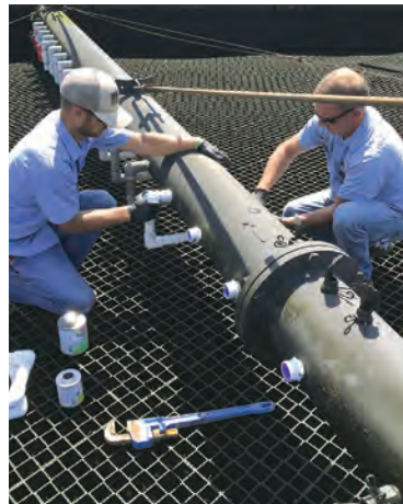
John Gaines, left, assistant superintendent, and Whit McCurley, mechanic, install 1.25-inch PVC pipe to distribute effluent behind the distribution arms.
