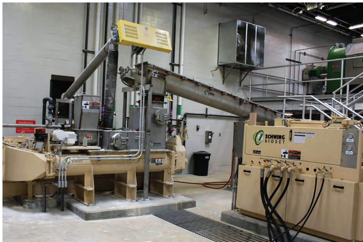
A screw conveyor takes untreated biosolids from the screw presses to a twin-screw mixer, where quicklime and sulfamic acid are added and mixed before being pumped to the reactor.
