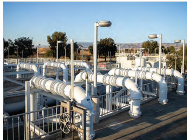
Mixed liquor return pumps recirculate nitrate as part of the denitrification process at the South County Regional Wastewater Authority in Gilroy, California.
