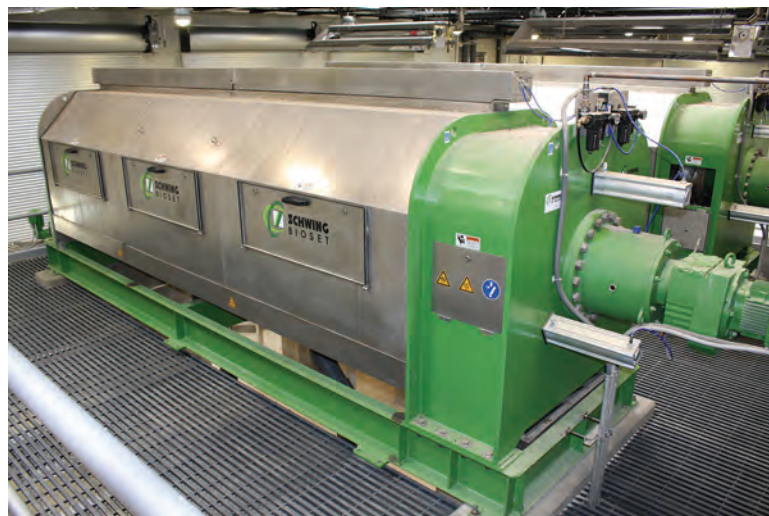
Each screw press is rated for 1,122 pounds of dry solids per hour, with a minimum 17% cake solids and a 95% minimum system solids capture. The presses continue to dewater during cleaning cycles so that no equalization storage is needed between dewatering and the Class A operations.
