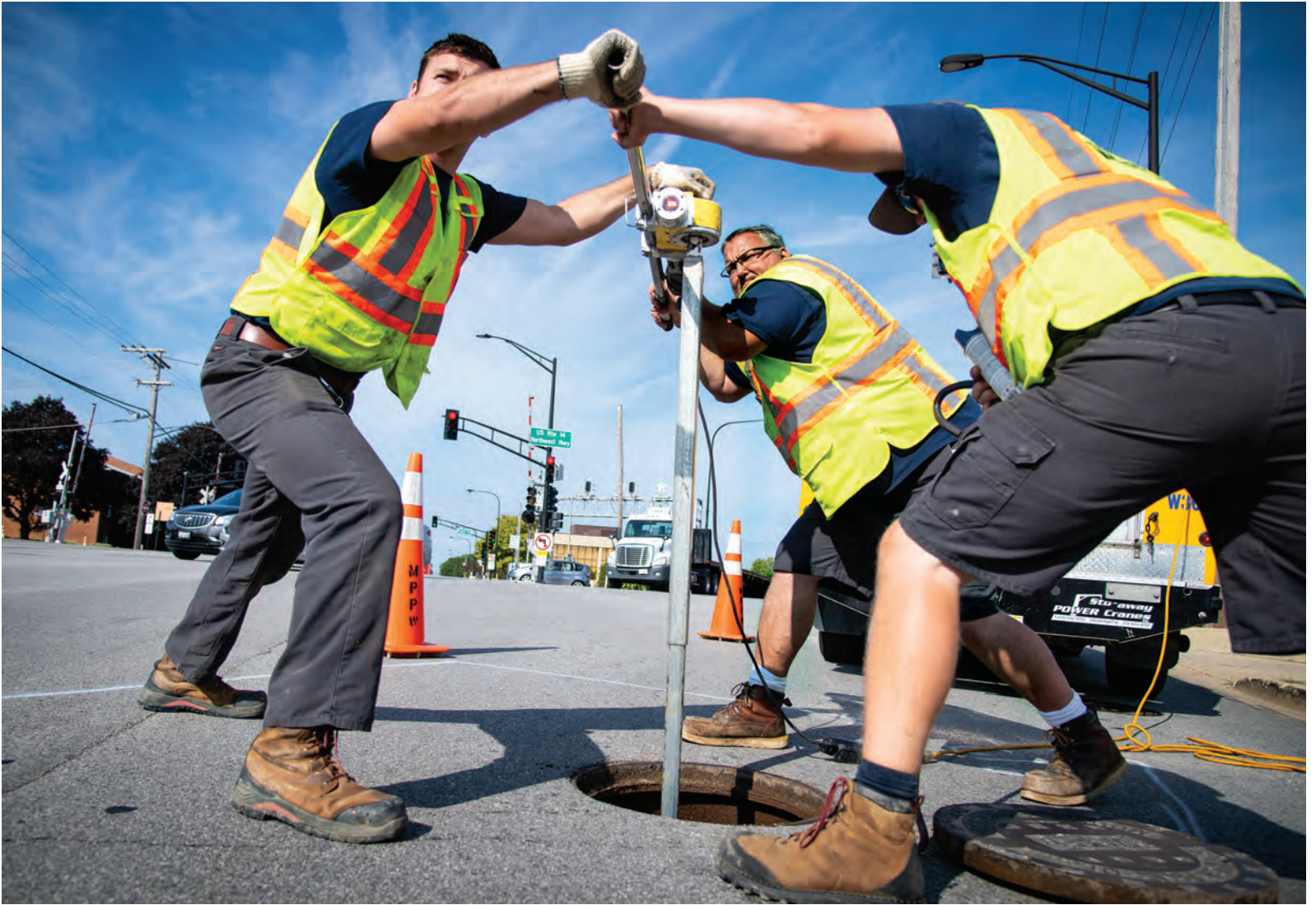
From right, maintenance workers Jake Sprow, Sean Feeney and Max Orlandi work on valve exercising, an important facet of the Mount Prospect distribution system maintenance program.
