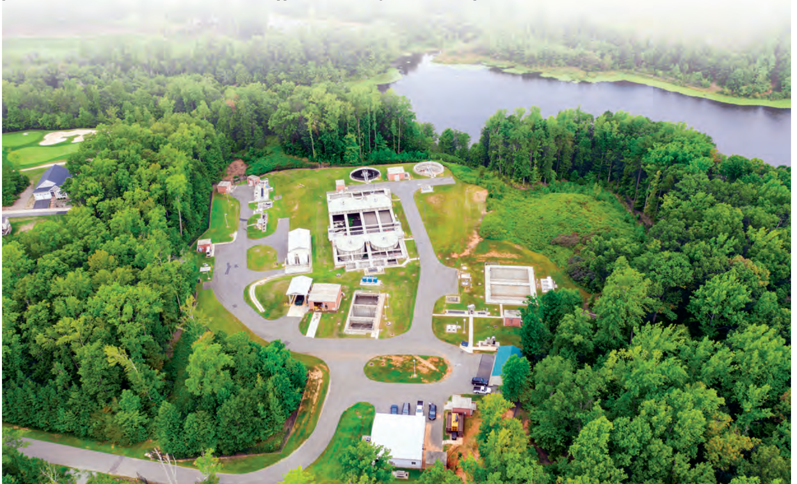
Aerial view of the Zion Crossroads Wastewater Treatment Plant.
