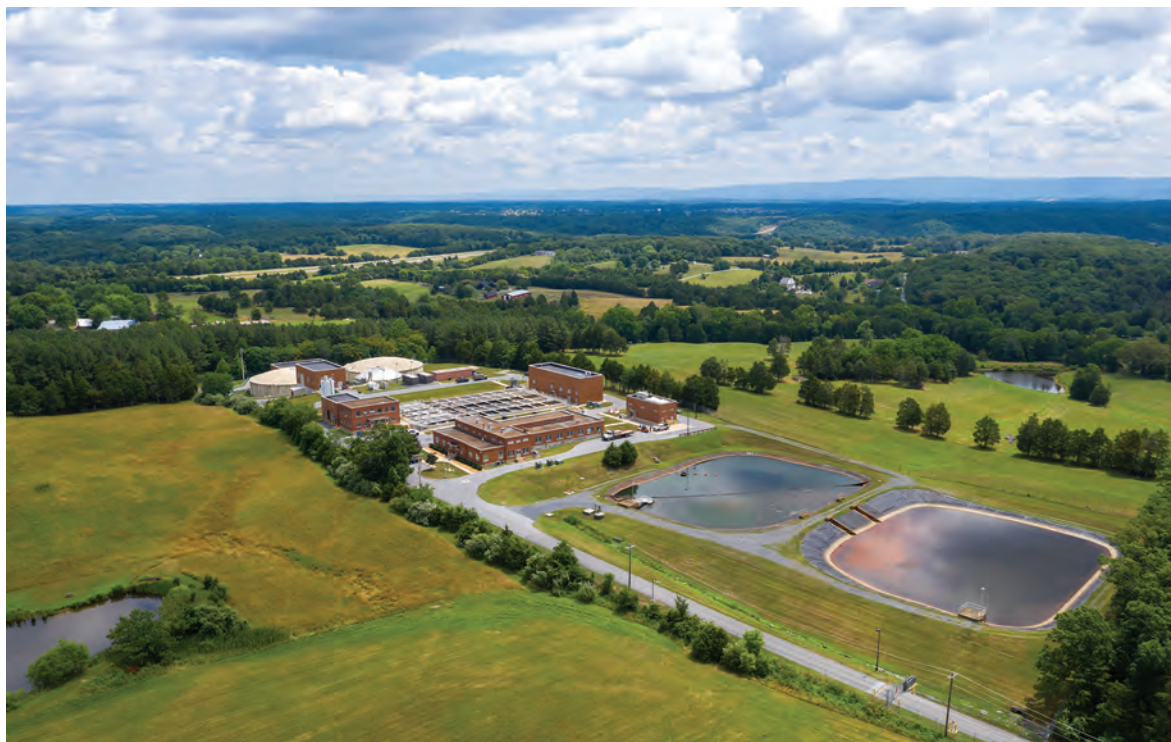
The Percy D. Miller Water Treatment Plant has a design capacity of 10 mgd.
