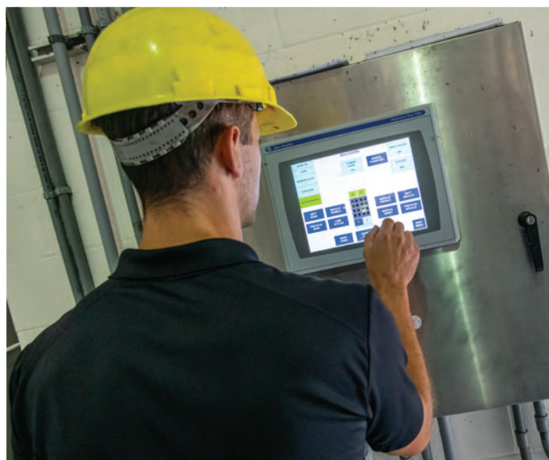
Callahan checks the status of the TrojanUV4000Plus (TrojanUV) disinfection system.
