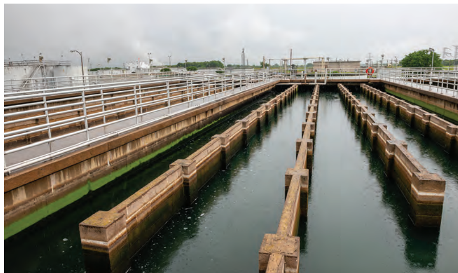
Effluent is disinfected in a chlorine contact basin before discharge.
