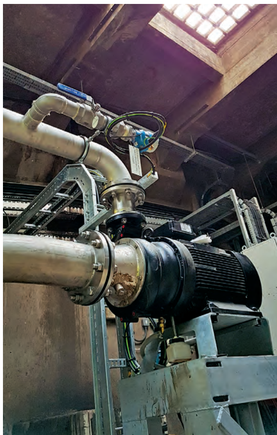
LEFT: Richard Thomson of MWH Treatment was instrumental in designing the chopper pump application. ABOVE: The Landia chopper pump provides continuous maceration of rags and debris.
