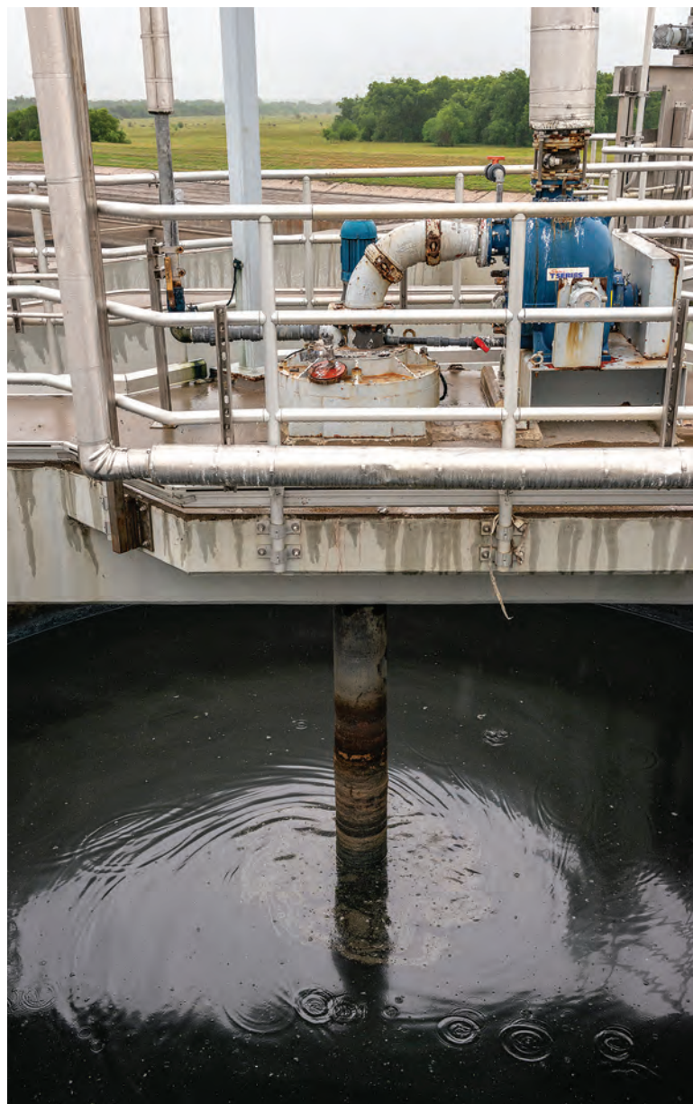
Circular flow created by the pump (Gorman-Rupp) in the grit basin helps filter sediment from the wastewater.
