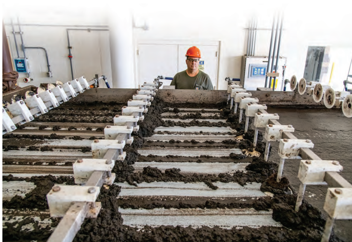
Matt Mink checks biosolids consistency in the gravity belt filter press (Komline-Sanderson) at the Bloomington-Normal Water Reclamation District Southeast plant site.
