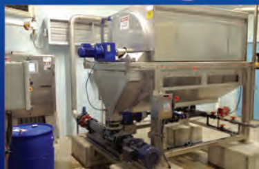
Rotary Drum Thickener
