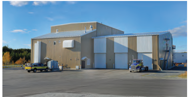
The biosolids facility transforms solids from all wastewater treatment plants in Greater Sudbury into Class A biosolids. The facility is owned by the city but operated by N-Viro and uses a patented N-Viro process. The final product is used in mine reclamation.
