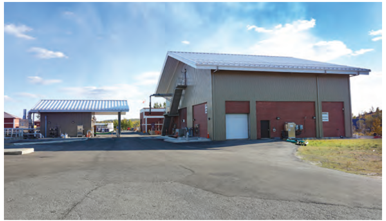
The receiving facility accepts solids produced at outlying wastewater treatment plants. The material is thickened from 0.5% to 3% solids before being sent to the biosolids facility for processing.
