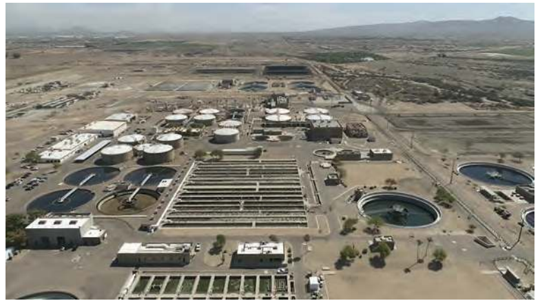
An aerial view of the 91st Avenue Wastewater Treatment Plant
