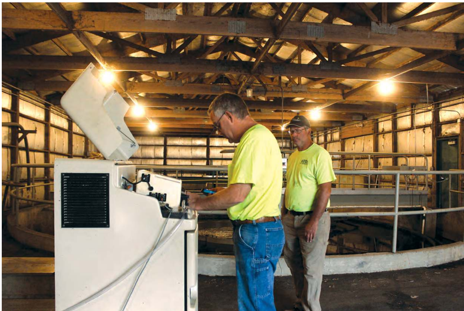
One of the two samplers at the Eagle River Wastewater Treatment Plant in Eagle River, Wisconsin. Daryl Rutkowski is turning on and checking over the sampler.
