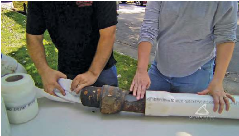
A video on the website shows a plumber inserting a liner into an old steel pipe while a collections system worker looks on and asks questions about the installation.
