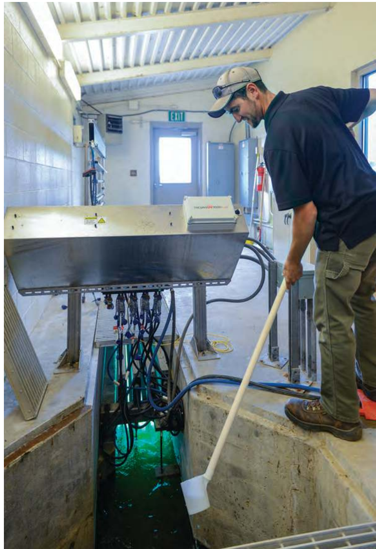
Mike Murphy takes an effluent sample to check the pH in the UV disinfection treatment phase (TrojanUV3000Plus).
