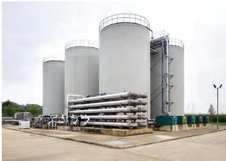
Biological hydrolysis increases hydrolysis efficiency by adding six serial reactor vessels in front of an anaerobic digestion system.
