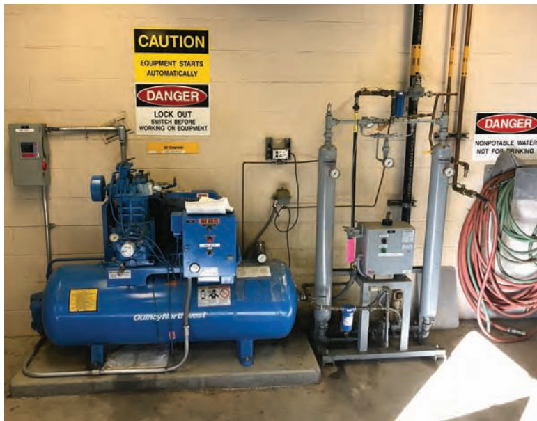
One project replaced this 40 hp compressor with a lower-powered unit, achieving a payback of six months from energy savings.
