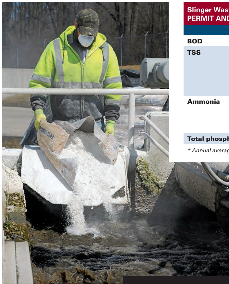
Joe Kell adds lime to the oxidation ditch twice a day as another technique for phosphorus reduction.
