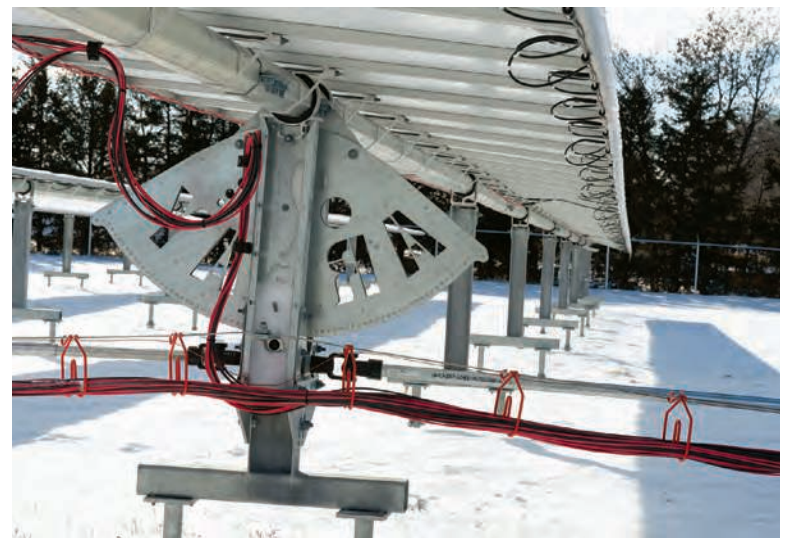
The panels are mounted on a mechanism that enables them to maximize exposure to sunlight through the day, boosting energy production by about 30%.
