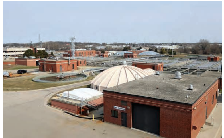
The Madison Metropolitan Sewerage District serves 26 customer communities covering 184 square miles and a population of 380,000.
