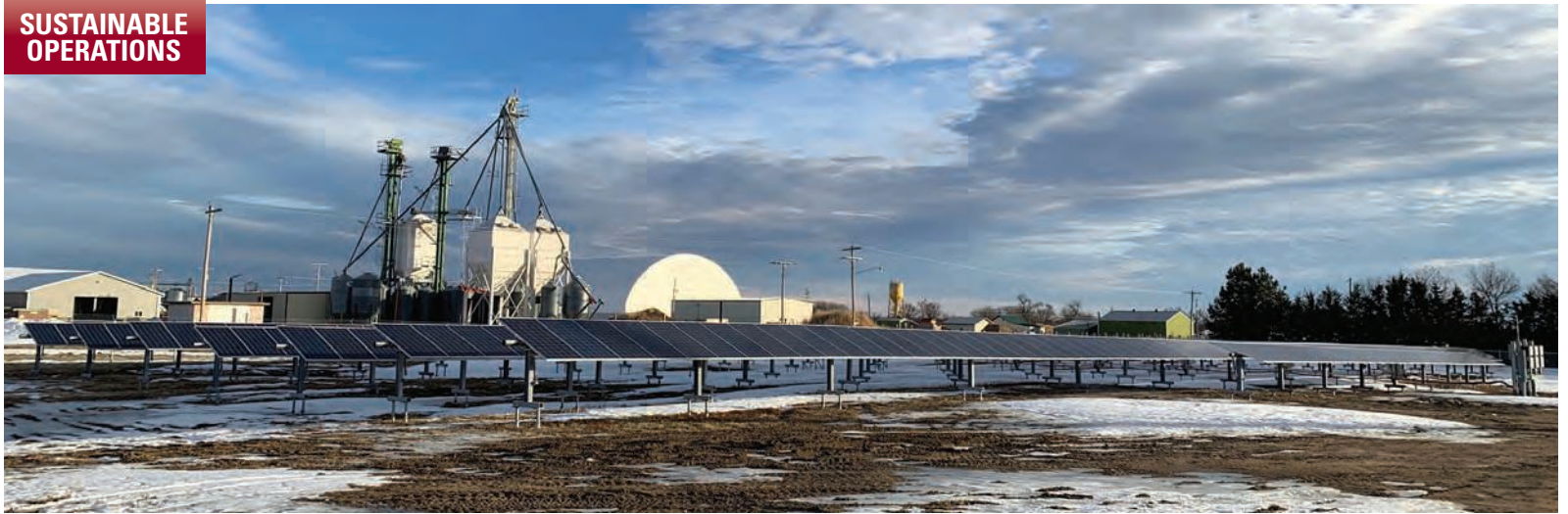
The solar array includes 668 panels and is expected to produce 377 MWh per year.
