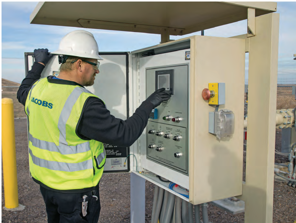
Kent Mindy with the thermal oxidizer that burns off impurities separated from the gas during the refining process.
