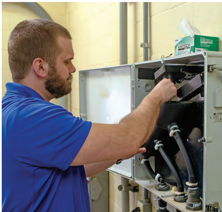
Gohman cleans the Hach Surface Scatter 7 sc turbidimeter.
