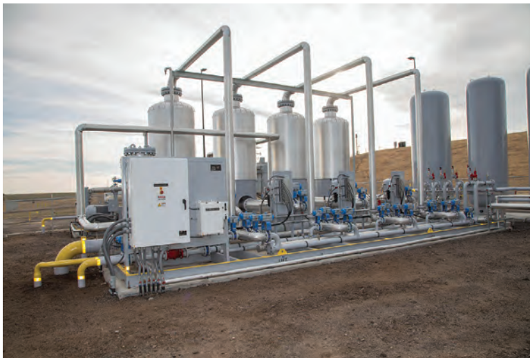
The Molegate skid (Guild Associates) filters raw gas in proprietary media.
