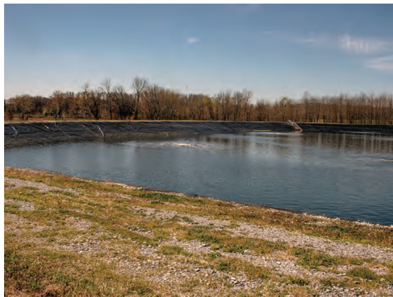
A 3.25-acre retention lagoon helps the Humboldt team manage high-peak flows caused by I&I.
