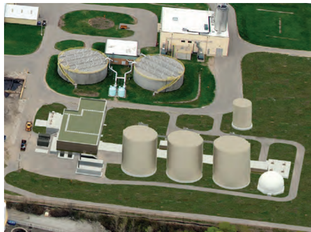
An artist's rendering shows the Grand Rapids biodigestion facility, which is under construction. The three digesters are the cylinders in the foreground.
