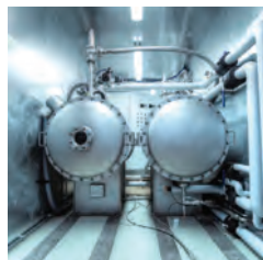
Capital Controls ozone generators from De Nora Water Technologies
