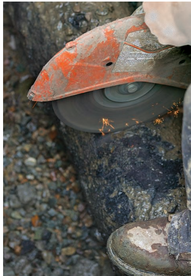
A saw is used to cut through an old water main.
