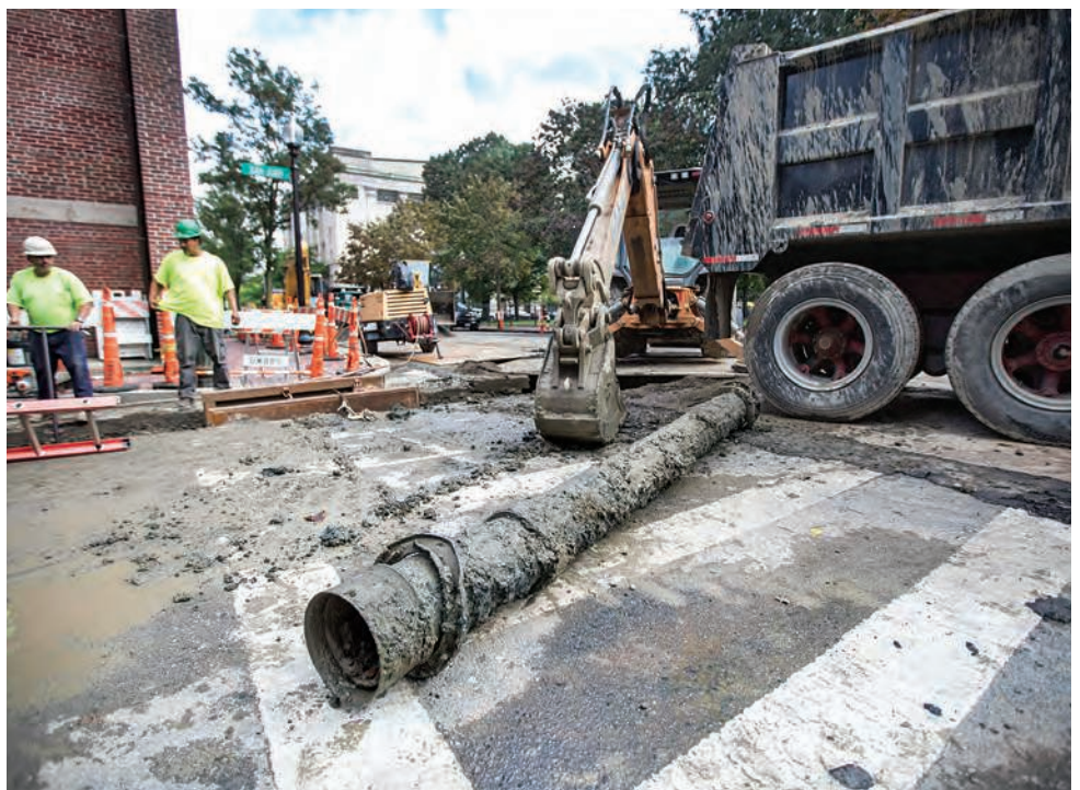
An old water main is shown after replacement by contractors.
