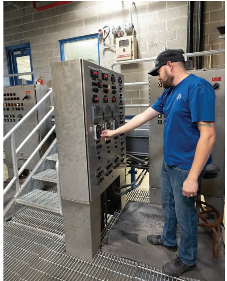
RIGHT: Dan Shorten adjusts the dosing of polymer (SNF Polydyne) in the press room. BELOW: Shorten, shown drawing a sample for analysis, is proud of how his team maintains the plant’s dewatering presses.
