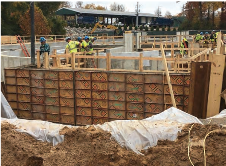
The closed-loop reactor at Ole Miss is shown during construction.
