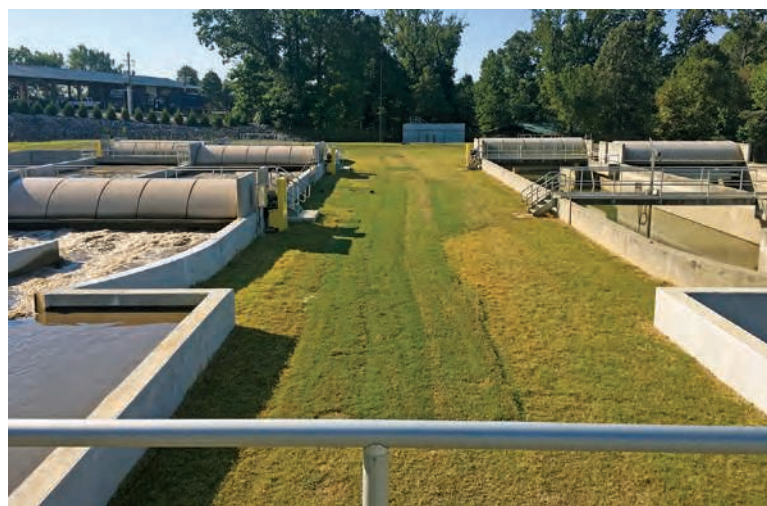
Original closed-loop reactor on the left; new closed-loop reactor on the right.
