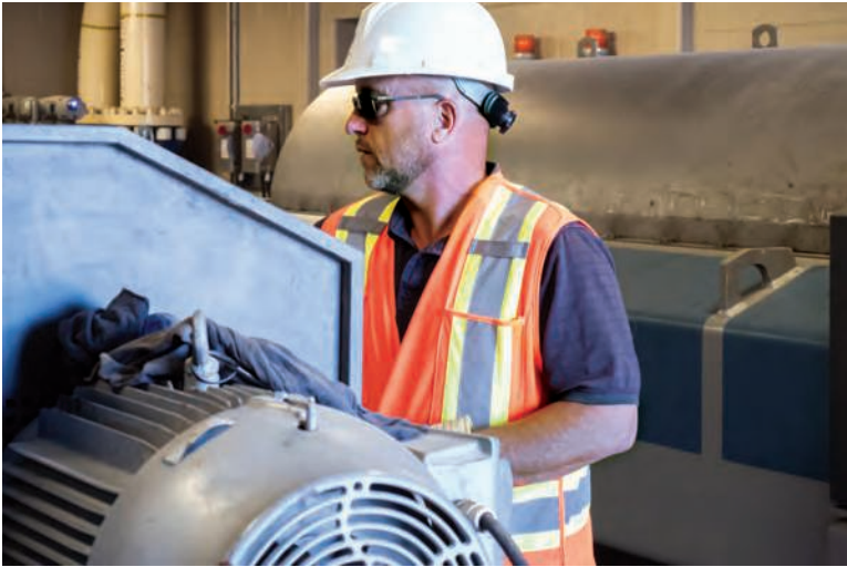
To optimize centrifuge efficiency, operators tested different polymer concentrations, feed rates and torque settings.
