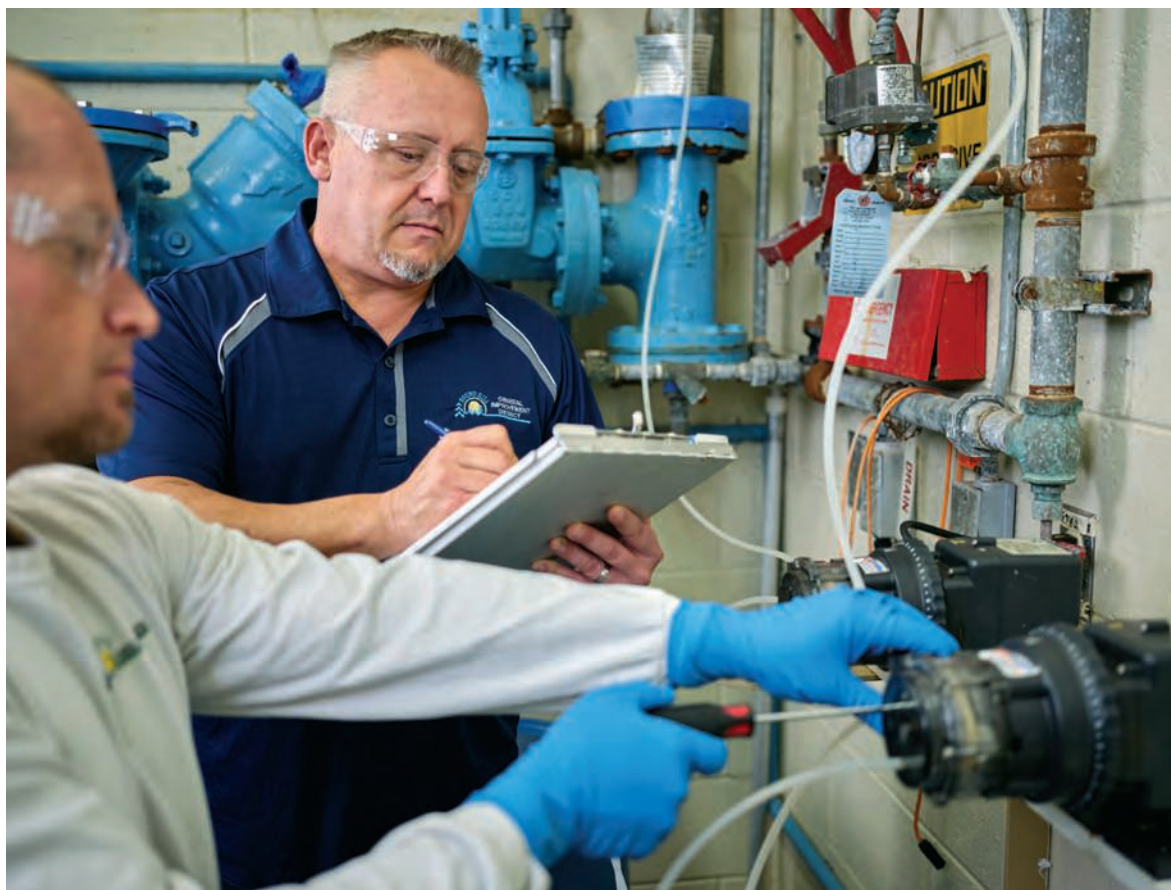
Andy Hickman observes operator Josh Bisset as he performs maintenance on a Stenner Classic Series peristaltic metering pump.
