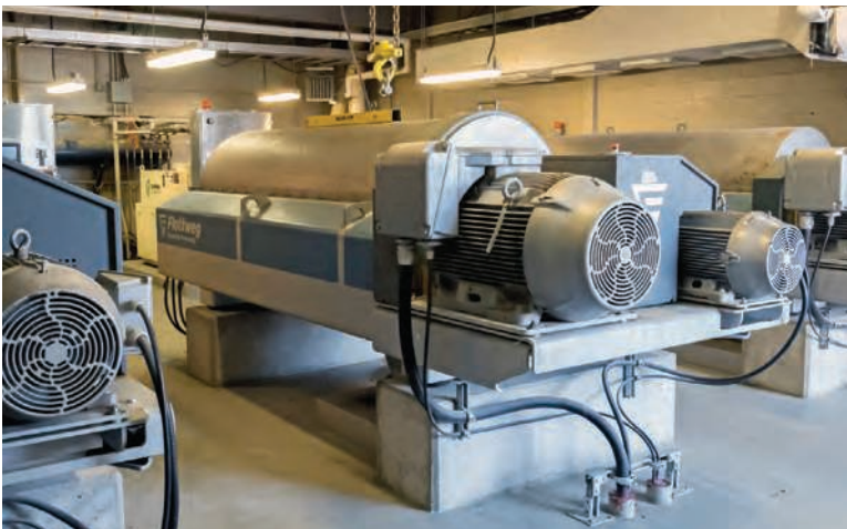
The centrifuges deliver biosolids cake at 26 percent cake solids and operate cost-effectively.
