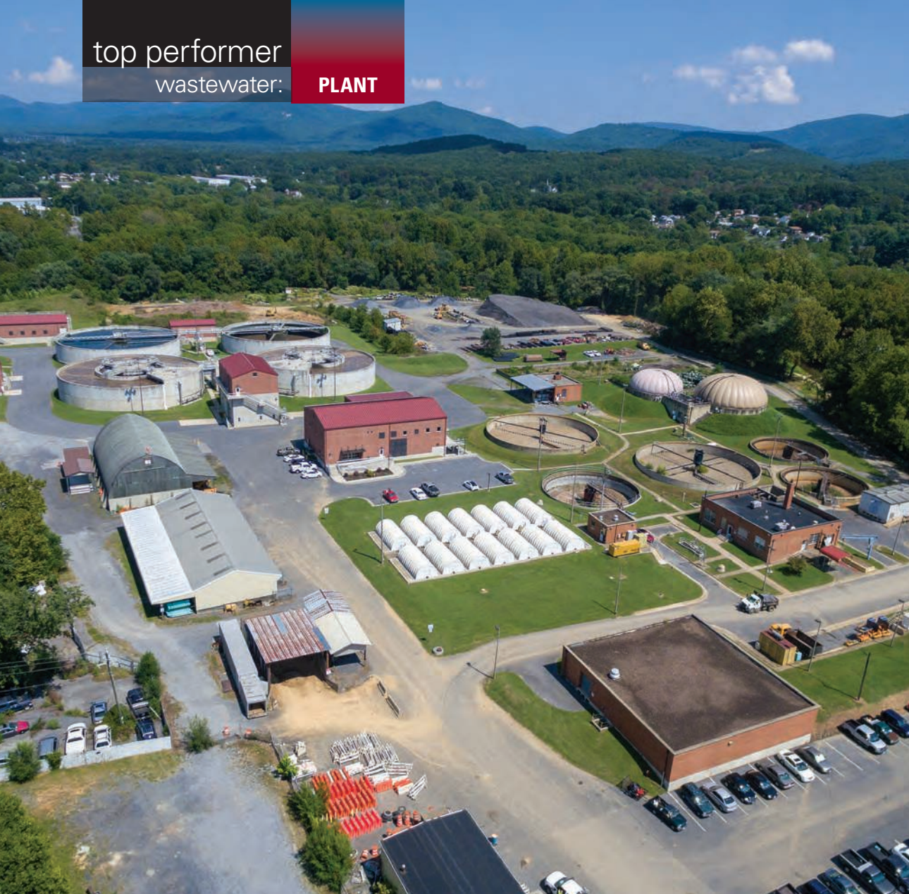
The City of Waynesboro wastewater treatment and water treatment plants.
