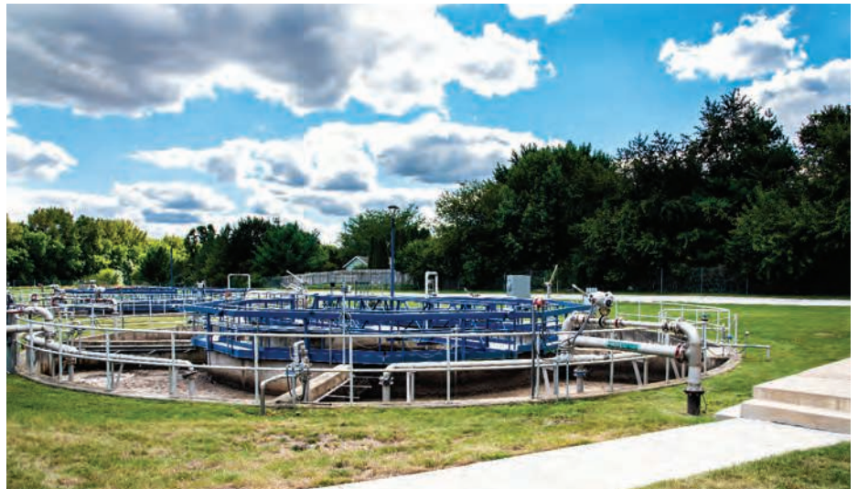
The Mahomet facility produces effluent containing monthly averages of 6.15 mg/L nitrate and 0.63 mg/L total phosphorus.
