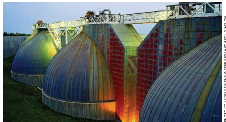
Co-digestion in digesters like these enables utilities to enhance energy recovery during wastewater treatment.
