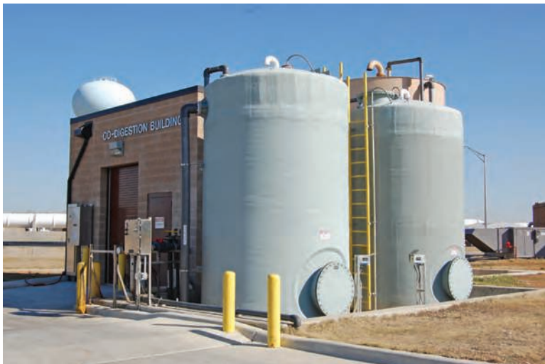
The co-digestion building facility received high-strength liquid food from a variety of sources.
