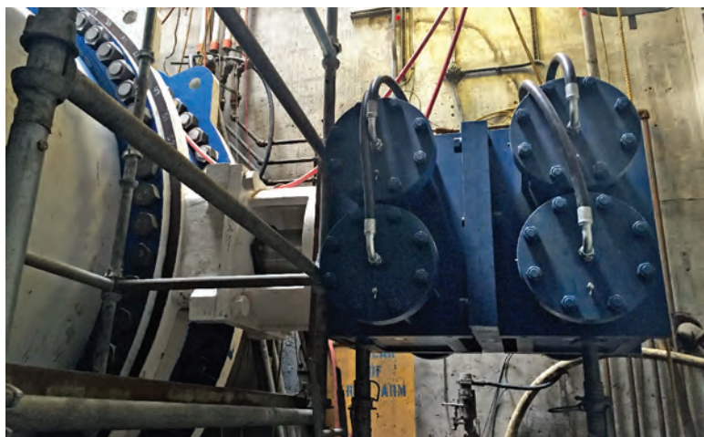
The newly installed 120-inch butterfly valve includes a dual Moog Flo-Tork actuator.
