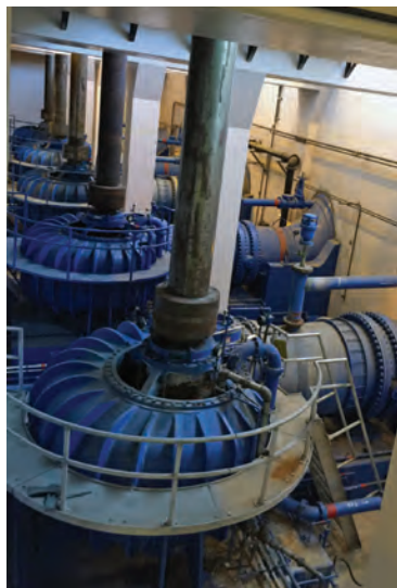
Deteriorating butterfly valves on the suction and discharge sides of these vertical turbine effluent pumps were refurbished.
