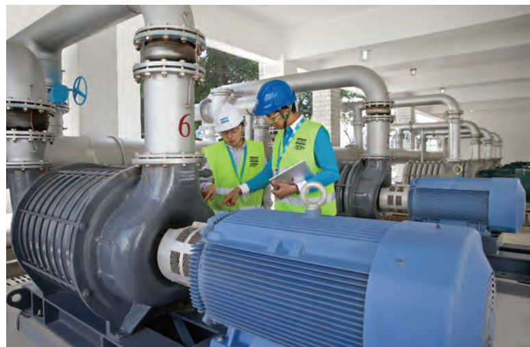
Indoor blower installations need to consider proper ventilation and effective heating or cooling to keep blowers operating within their temperature limits (Atlas Copco ZIM multistage centrifugal blowers are pictured).
