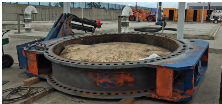
An old 120-inch butterfly valve with dual-cylinder operator was replaced as part of the valve upgrade project.
