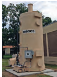
HIBOCS odor control vessel from Heyward Florida
