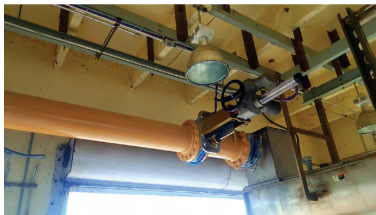
Cake discharge into an existing overhead conveyor.
