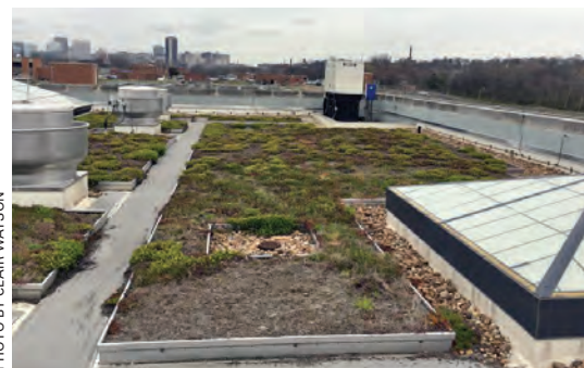
A winter view of the 2,400-square-foot green roof on the wastewater treatment plant's UV disinfection building.
