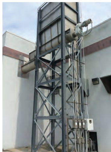
The original vertical conveyor at the Glades Wastewater Treatment Facility.
