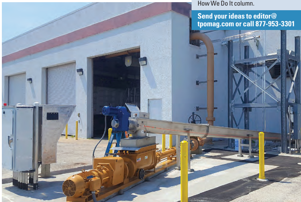
LEFT: Tight spaces below the existing centrifuges. BELOW: New biosolids cake pump installation (SEEPEx).
