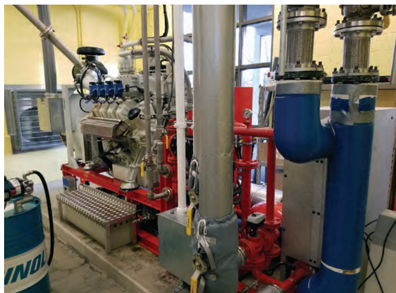
One of the two biogas-fueled engine-generators (Nissen) that form the heart of the combined heat-power system.
