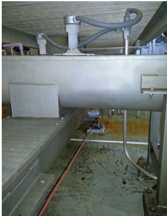
LEFT: Tight spaces below the existing centrifuges. BELOW: New biosolids cake pump installation (SEEPEx).
