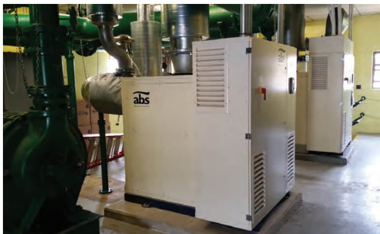
High-speed turbo blowers replaced older blowers at the Downers Grove plant (Sulzer Pumps Solutions).
