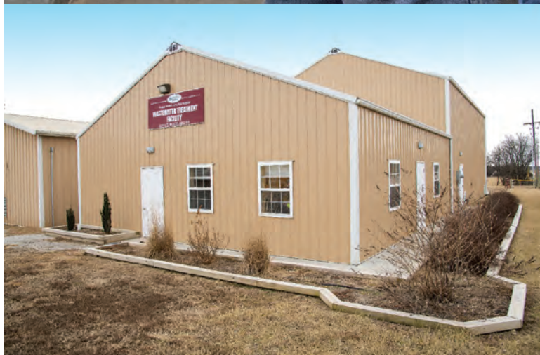
The main office building at the Spring Hill water treatment plant.
