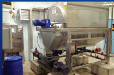
Rotary Drum Thickener
