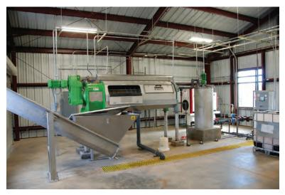
The plant upgrade included replacement of plate presses for solids dewatering to a screw press (Schwing Bioset) that occupies less space and saves on labor.
