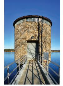
The new stone tower intake structure encloses the intake pumps providing security and keeping their operation quiet.
