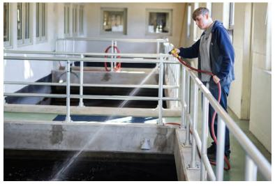
Christopher Litteral works in the filter room, equipped with sand, anthracite, and gravel filters and an underdrain system from Leopold, a Xylem brand.
