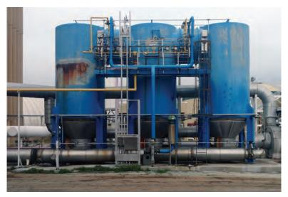
Three regenerative thermal oxidizers remove odors and pollutants from biosolids dryer emissions at JEA.
