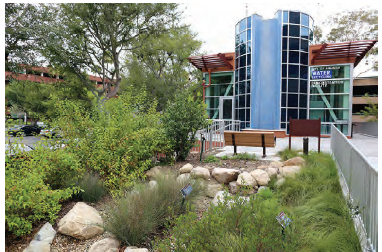
The Anaheim Water Recycling Demonstration Facility produces 100,000 gpd of water for landscape irrigation.
