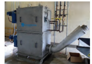
ProTechtor Centerflow Band Screen from Kusters Water, division of Kusters Zima Corp.
