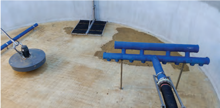
The Moore County Wastewater Treatment Plant SBR aeration tank before filling (above), and in operation (below).
