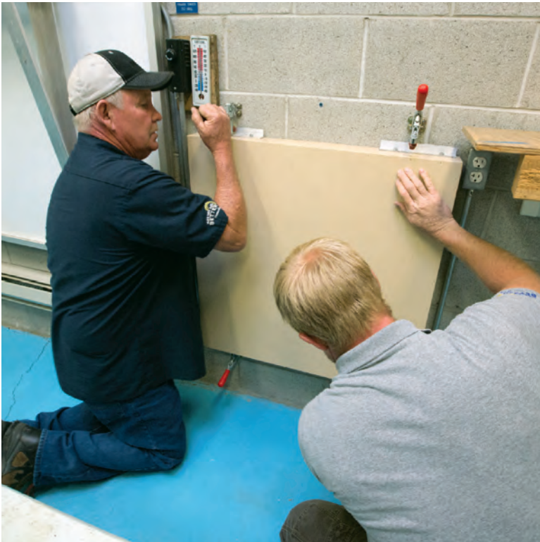
ABOVE: A Reliance Super-E Motor (Baldor Electric) operates at a lower pressure than is traditional. It pumps water in circles to keep the system pressurized, saving utility demand charges. BELOW: Ron Blackman and Steve Hunt install an insulated vent cover to conserve heat and save energy at the Church Well fill station.
