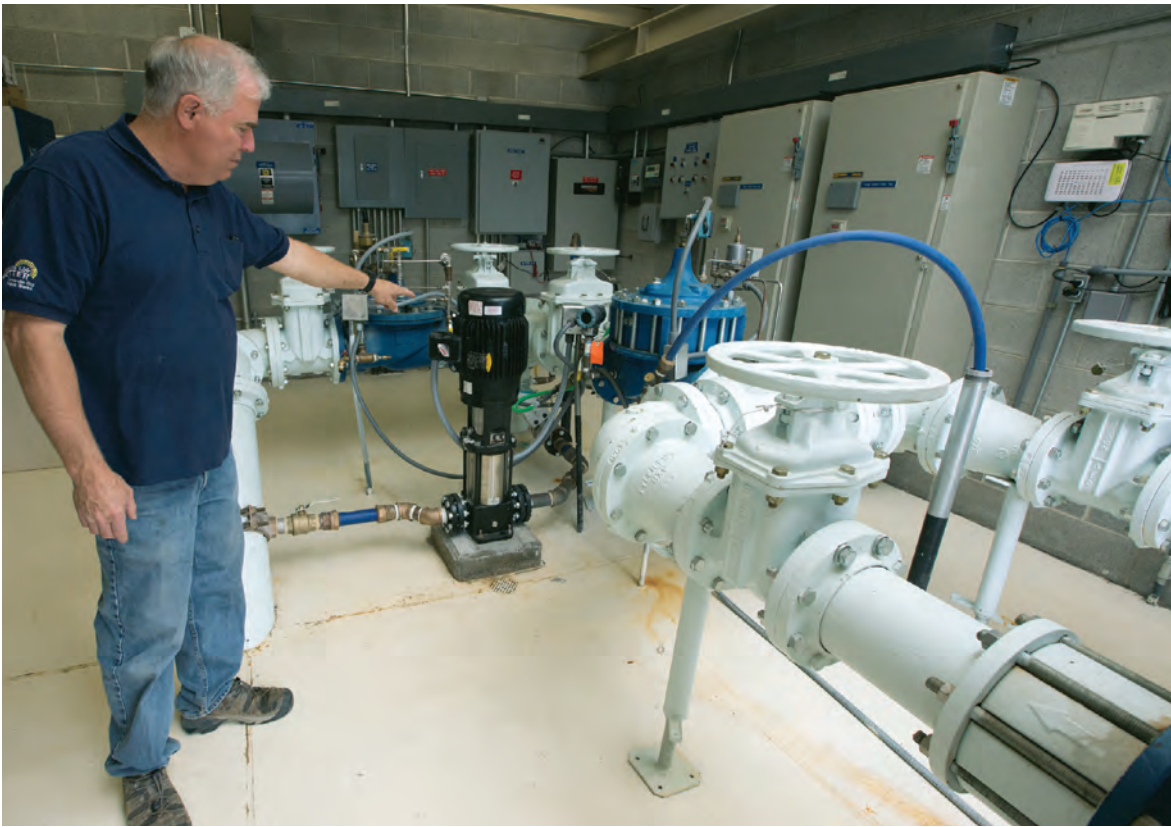
ABOVE: A Reliance Super-E Motor (Baldor Electric) operates at a lower pressure than is traditional. It pumps water in circles to keep the system pressurized, saving utility demand charges. BELOW: Ron Blackman and Steve Hunt install an insulated vent cover to conserve heat and save energy at the Church Well fill station.
