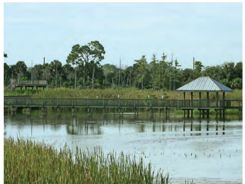
The boardwalk spans one-half mile and includes a covered pavilion.
