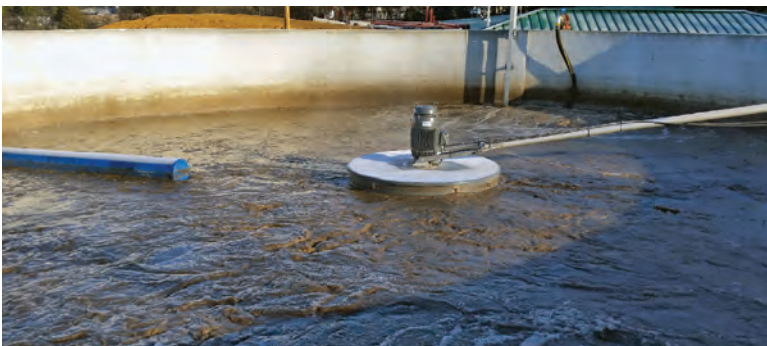
The Moore County Wastewater Treatment Plant SBR aeration tank before filling (above), and in operation (below).
