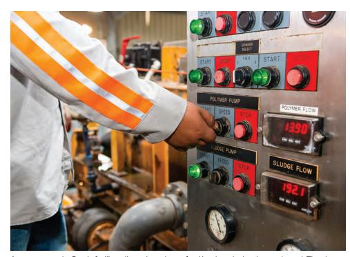
An operator at the Renda facility adjusts the polymer feed levels at the local control panel. The plant lowered polymer usage by about 30 percent, helping to reduce odor complaints.
