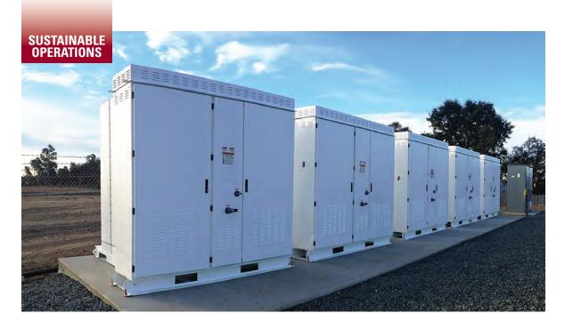
The battery system supplied by Tesla is rated at 1 MW/2 MWh and so could discharge 1 MW for two hours or a smaller amount for more time. The project cost \$3.2 million.
