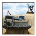
**Emergency Vent and** Pressure/Vacuum Vent and Flame Arrester
