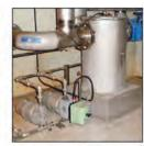
Sediment Trap with **Electrically Actuated** and Manual Drip Traps
