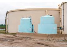
Chlorine dioxide tanks (blue) stand in front of the liquid storage tanks (tan).
