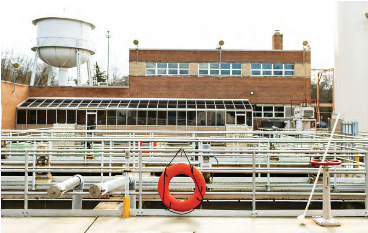
Carlisle Borough Water Treatment Plant produces an average of 2.5 to 3 mgd for distribution through 77.2 miles of mains.
