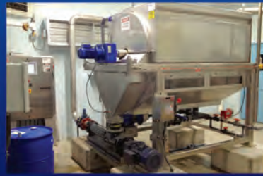
Rotary Drum Thickener
