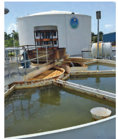
One of two lime softening accelerators. A 2-million-gallon storage tank appears in the background.
