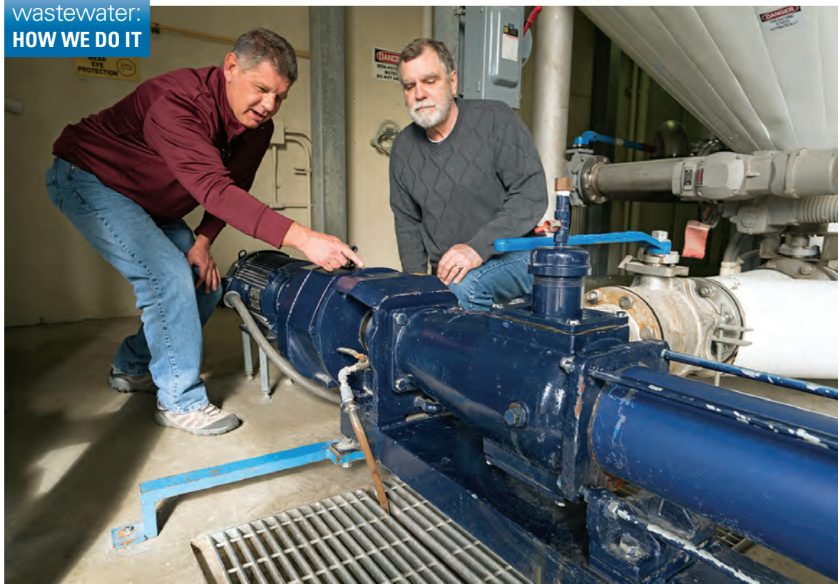
Jordan Kleinsmith, assistant plant manager, and Craig Carter, plant manager, with one of several progressive-cavity pumps used in multiple applications in the Carmel treatment facility.
