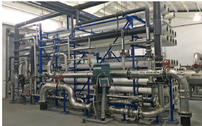
The plant design pushed the envelope with a fourth stage in its nanofiltration membrane systems (Hydranautics).
