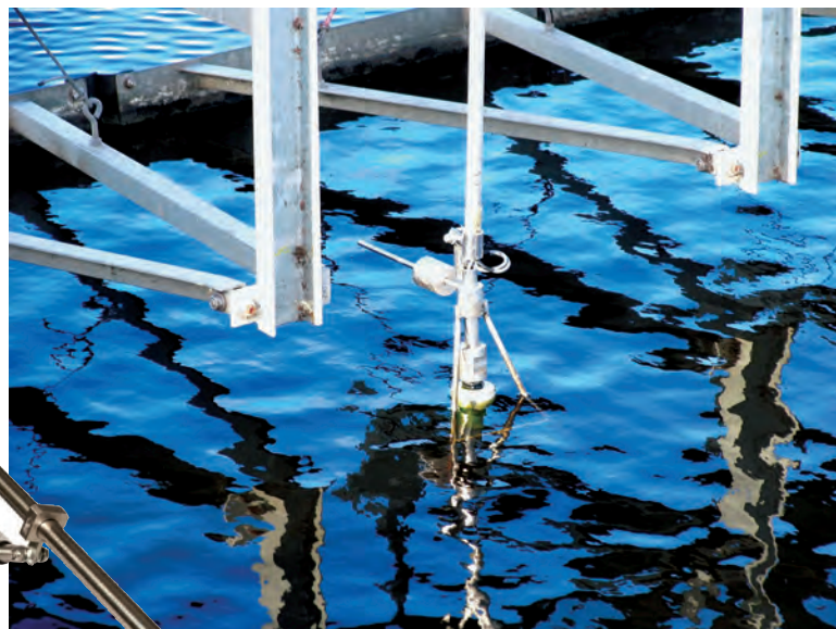
An ORCA sonar system (Hawk Measurement) is shown in full profile and as mounted to measure sludge levels in a clarifier basin.
