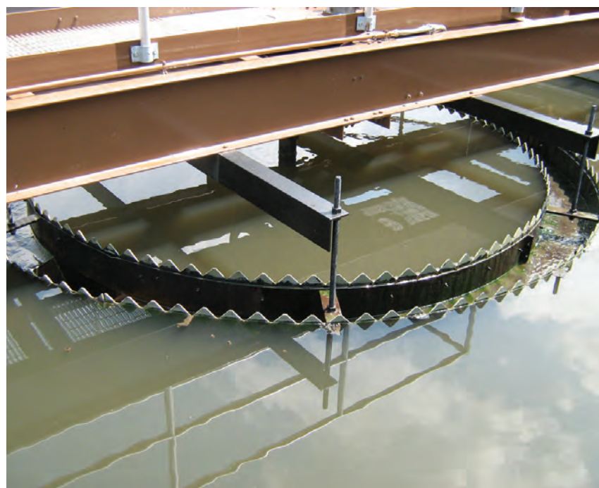
The new Spiraflo clarifier at the Addison Village plant (Lakeside Equipment Corporation).
