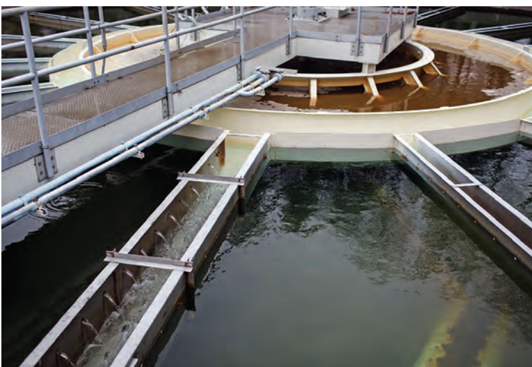
The turbidity of raw water coming from the Glendola Reservoir ranges from 2 to 5 NTU. The water leaves the plant at 0.1 NTU.
