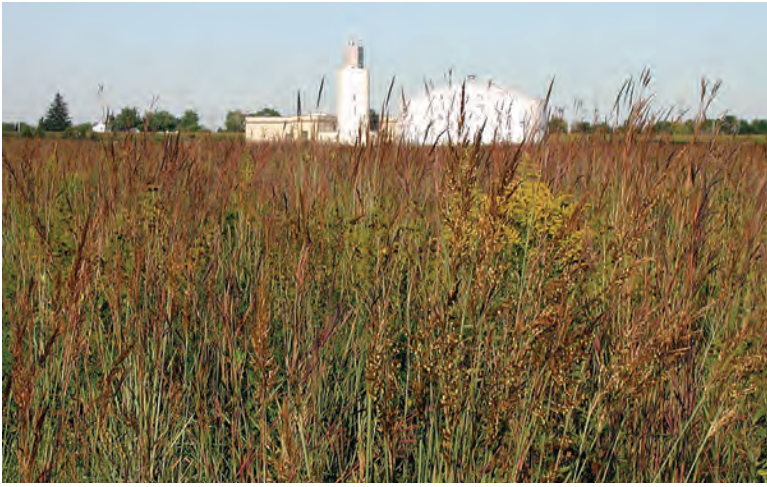
The constructed grassland with the Phillips Street Water Treatment Plant shown in the background.
