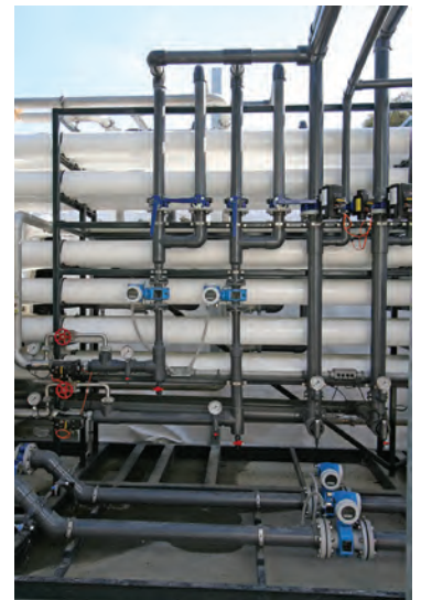
The plant's reverse osmosis system (Wigen Water Technologies).
