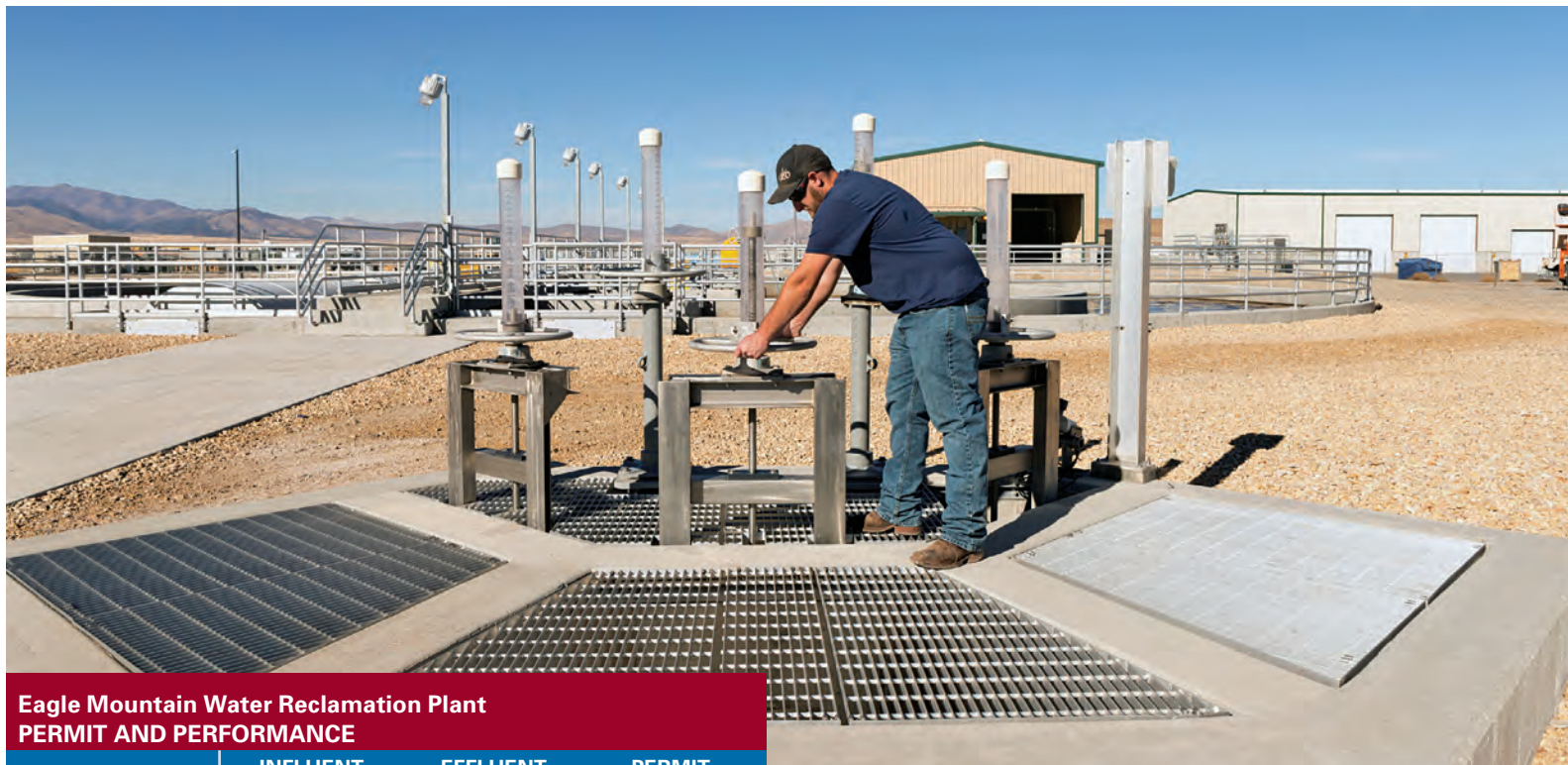
Dalton Harris checks the splitter box.
