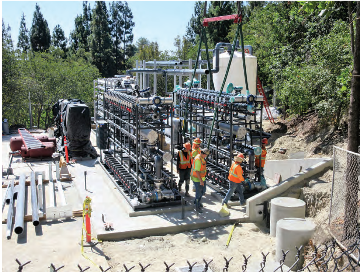
Workers place the facility's ultrafiltration skids.
