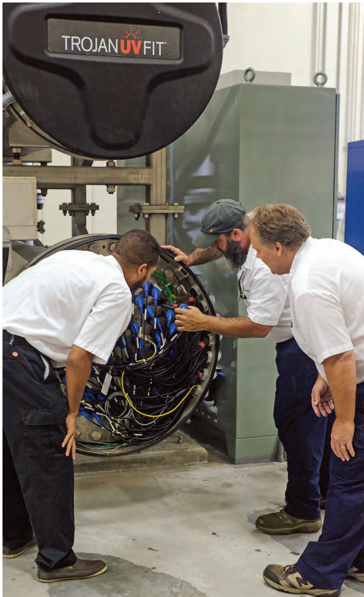
From left, plant operators Walter Fletcher, Todd Tysinger and Scott Hull inspect connectors on the TrojanUVFit disinfection unit.
