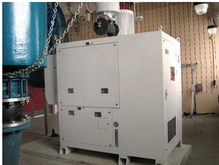
A single 350 hp high-efficiency turbo blower (APG-Neuros) now does the job of two fixed-speed 200 hp blowers and saves about $56,400 a year.
