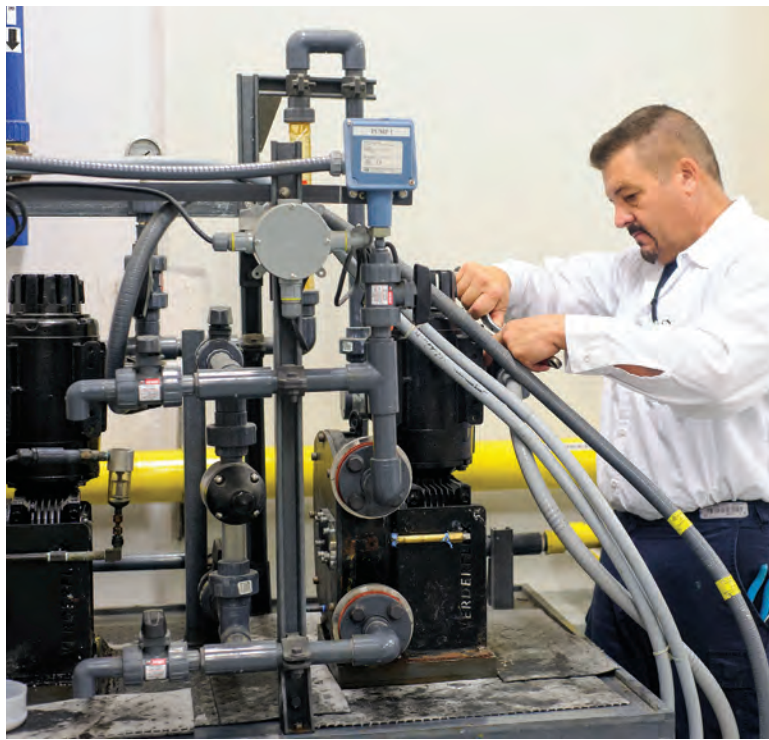
Greg Cavicchia performs maintenance on a Verderflex Dura 25 peristaltic pump chemical feed system (Verder).
