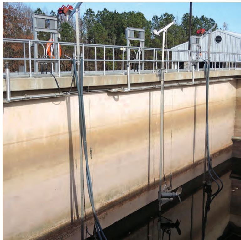
Landia submersible mixers and air-jet units mix and aerate the biosolids sludge tanks at Durham County.
