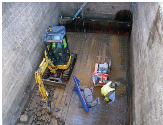
FIGURE 4. Left, demolition of a false-floor underdrain. Right, installation of a dual parallel lateral underdrain.
