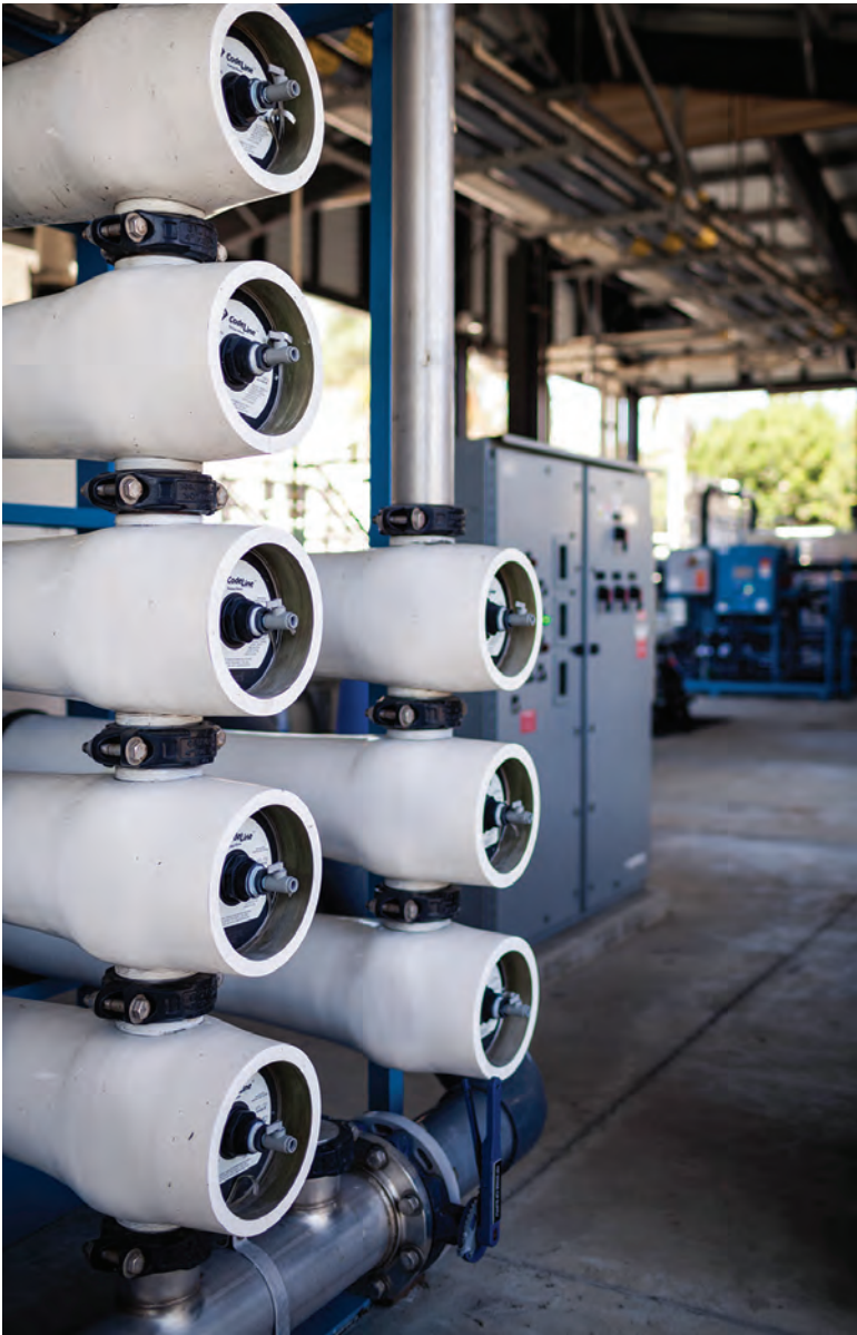
The water reclamation plant uses a combination of reverse osmosis (Water Equipment Technologies - a Xylem Brand), and microfiltration (Pall Corporation) in processing water from the upscale beach cities of Del Mar, Solana Beach and Encinitas.
