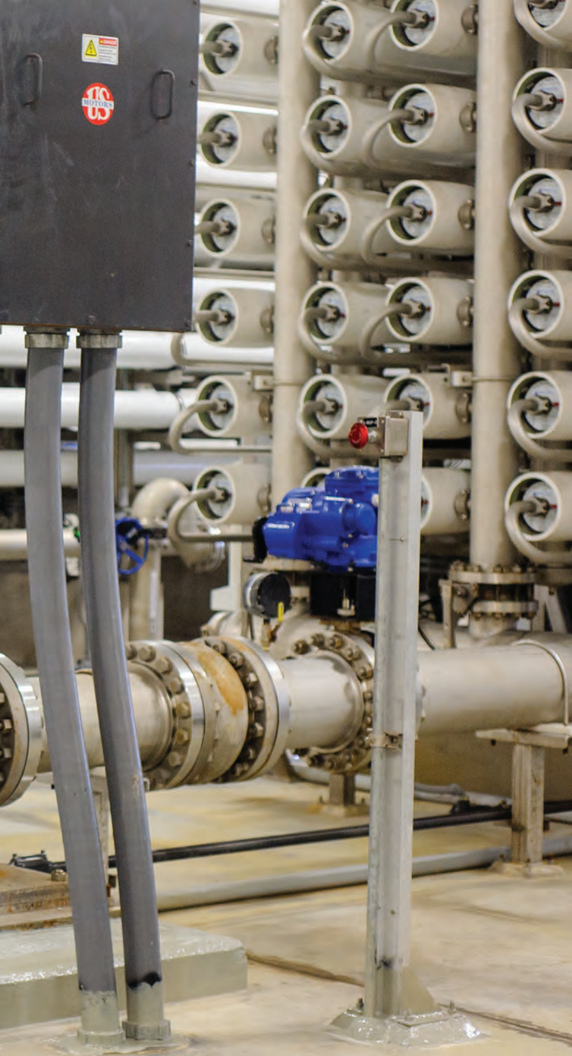
Plant mechanics Greg Cavicchia (left) and Tony Tristram inspect the reverse osmosis system at the Town of Davie Water Reclamation Facility. (Pumps by US Motors [Nidec Motor Corporation].)
