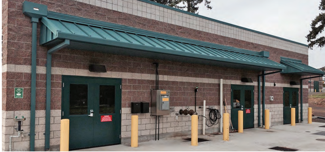
Hauling contractors deliver 70,000 gallons of FOG every week, allowing the Durham plant to run its cogeneration engines at full capacity.
