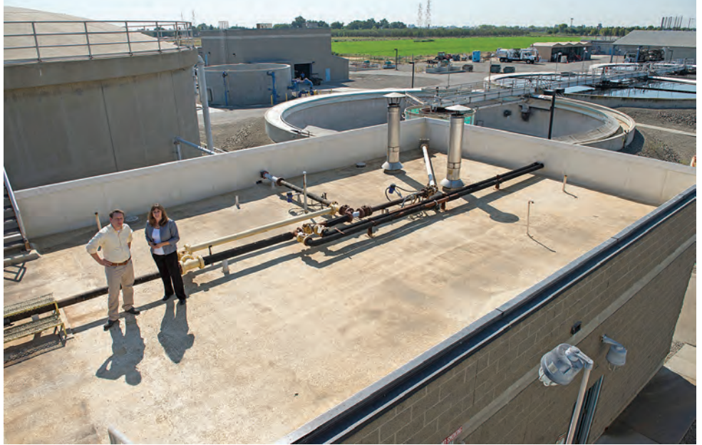
Manteca's $29 million food-waste-to-fuel project will include construction of receiving stations for food slurry and FOG, a control building, two digesters, gas compressors and fueling stations.
