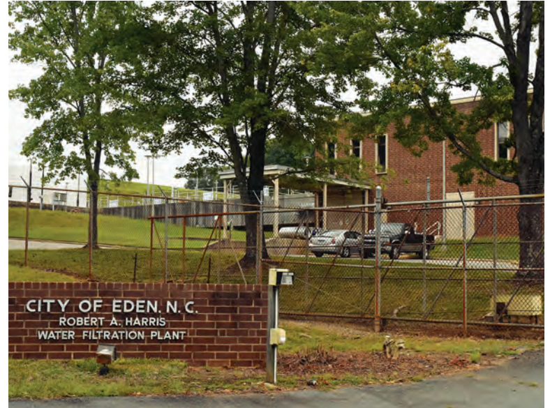
The water filtration plant in Eden has seven filters and two 4-million-gallon tanks that store water for customers. A lake behind the plant holds water taken in from upstream.
