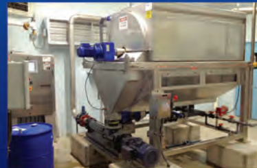
Rotary Drum Thickener
