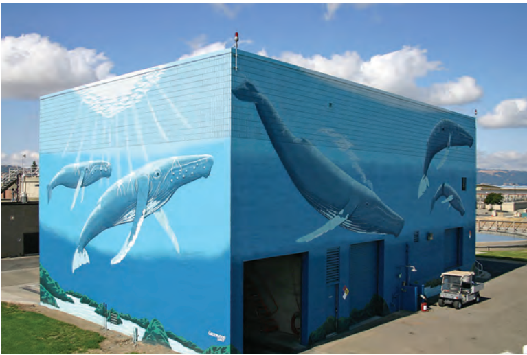
All four sides of the solids handling building show whales. A sandy ocean floor with coral outbreaks can be seen at ground level.
