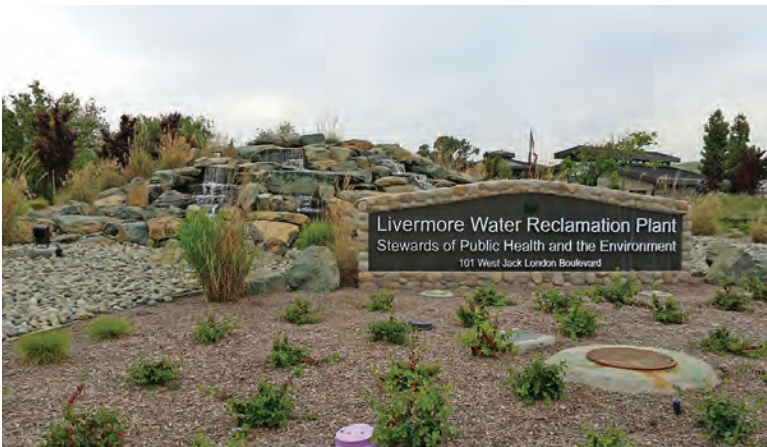
The waterfall feature and the new sign near the plant entrance were completed in 2015.
