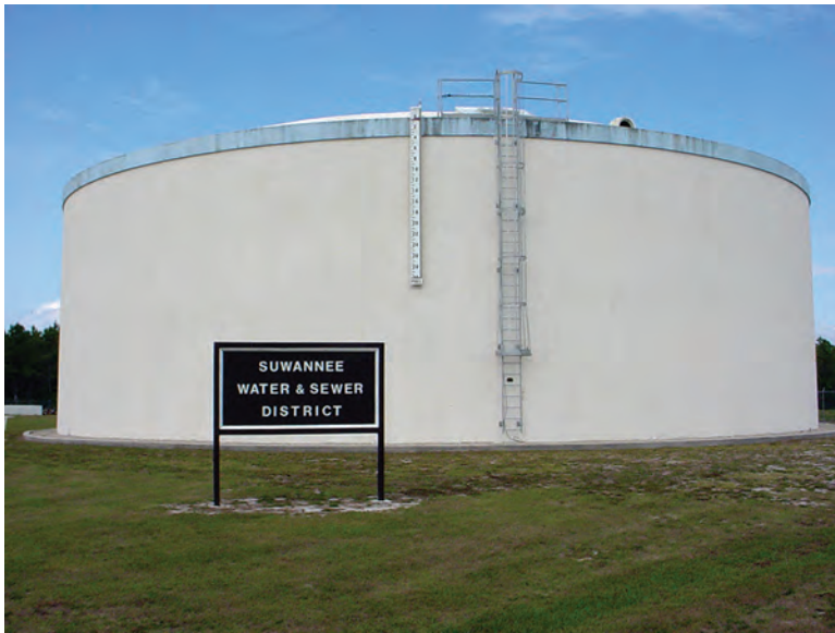
A digester at the Suwannee facility.
