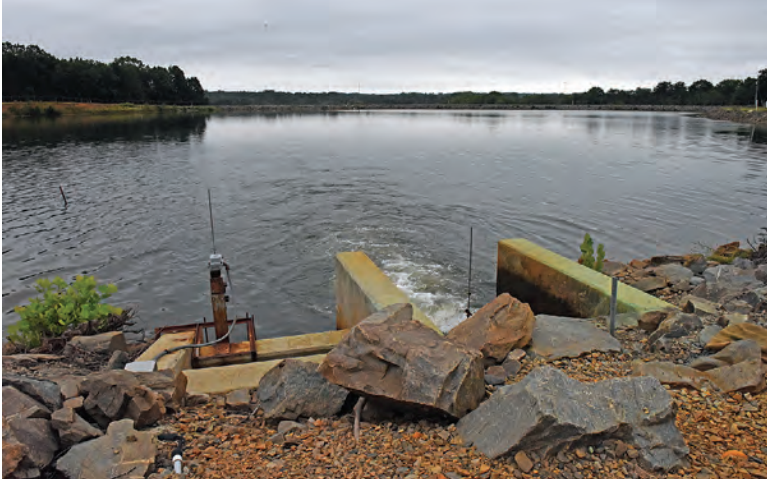
Source water is fed into a lake directly behind the filtration plant.
