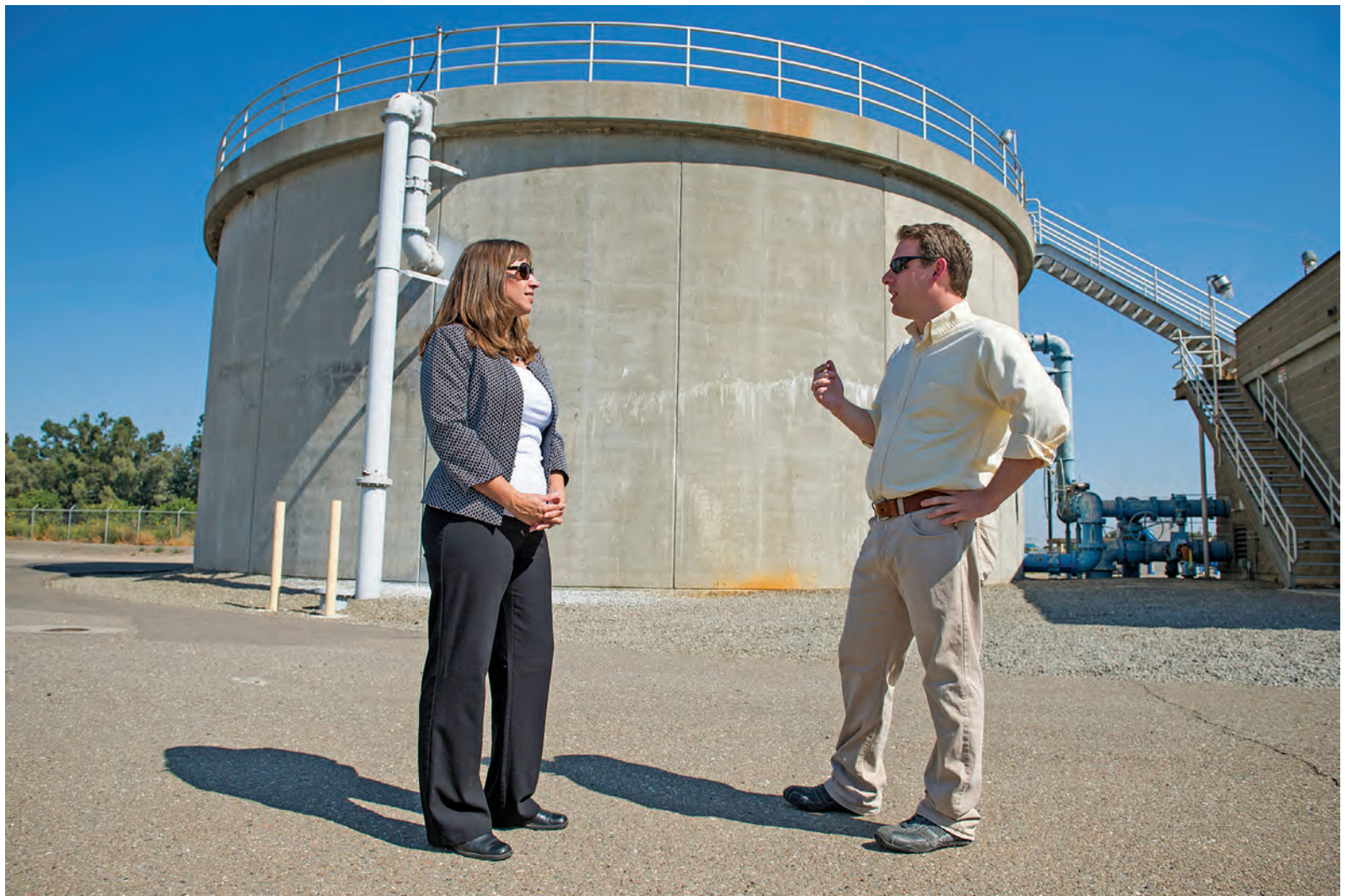
Heather Grove, wastewater system superintendent, and Jeremy Kline walk the wastewater treatment plant grounds where digesters will soon be updated as a step toward producing fuel for vehicles.
