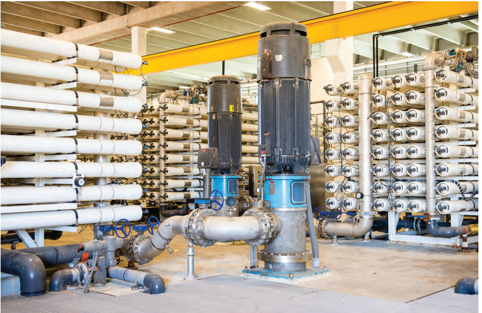
The reverse osmosis system at the Cypress Water Treatment Plant includes an impressive gallery of membrane modules.
