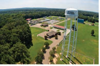
Shutting down one aeration basin helped the Wilako Wastewater Treatment Plant save \$70,000 a year on energy. Using two old lagoons to store inflow during heavy rains helped the plant deal with I&I issues.
