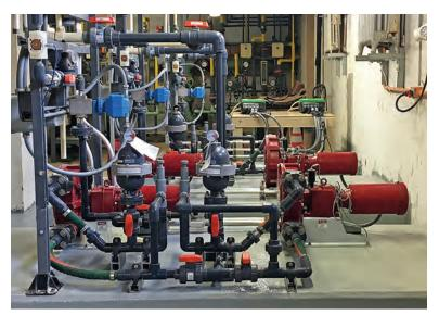
The Omohundro plant alum feed system, showing the feed pumps, pulsation dampeners, flowmeters, carrier water system, isolation valves, and pressure relief valves. Secondary containment was provided.
