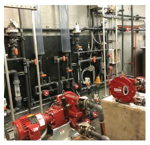
The Omohundro plant powdered activated carbon feed system delivers a slurry of 1 pound of carbon to 1 gallon of water. Each pumping system is designed while running to flush on a timed cycle to prevent sedimentation and blockage in the feed piping.
