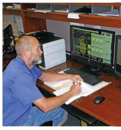
Don McIlhargey, chief operator, checks SCADA system readings and makes adjustments. While the plant is manually operated, the SCADA system tracks dissolved oxygen in the aeration basin, helping operators maintain proper levels.
