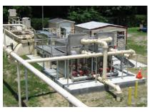
manufacture, installation, removal and maintenance, while maximizing treatment area. Media elements can be independently isolated and removed without discontinuing flow to the entire filter or diverting flow during routine maintenance or inspections.
