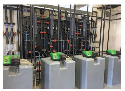
The Omohundro plant fluoride feed system, showing the feed pumps, carrier water system, isolation valves, and pressure relief valves. The system also includes a day tank with scale for accurate chemical dosing. Secondary containment was provided around the feed system.
