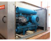
the control system is programmed to operate both blowers at two speeds without frequency converters. This means the total pumping speed may be set to four levels, saving energy. The control system runs the blowers for up to 12 hours a day. Control of dissolved oxygen is automated.
