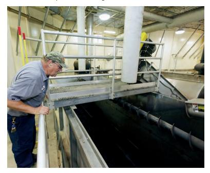
percent solids. A 15 hp blower pulls captured steam from the chamber through a duct as a spray of cool water condenses the steam. This water returns to the plant for treatment.
