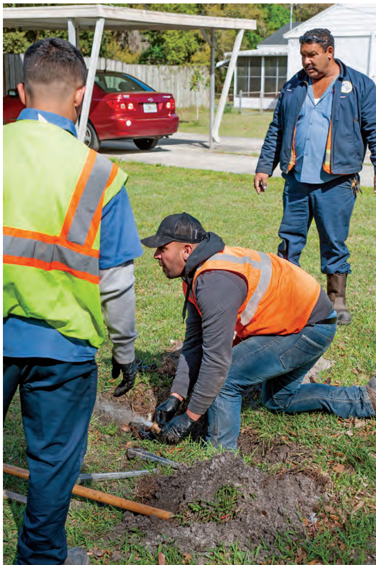
Team members from the Plant City utility connect HDPE tubing from a water main to a customer water meter. Pictured, from left, are David Velez, Luis Baez, and Victor Castro, maintenance specialists.
