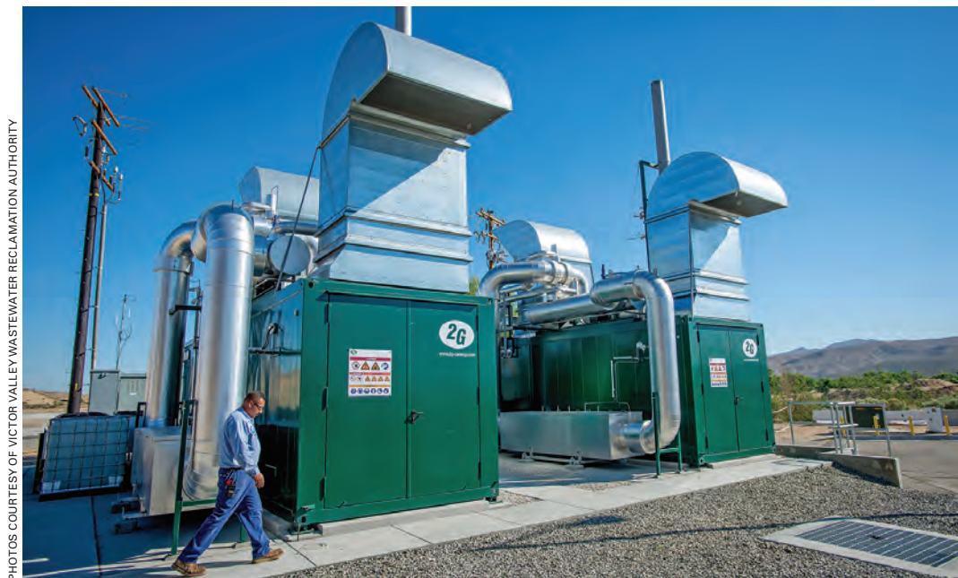
The Victor Valley Wastewater Reclamation Authority has two 800 kW engine-generators (2G Energy) fueled with biogas produced by the Omnivore anaerobic digestion system (Anaergia).
