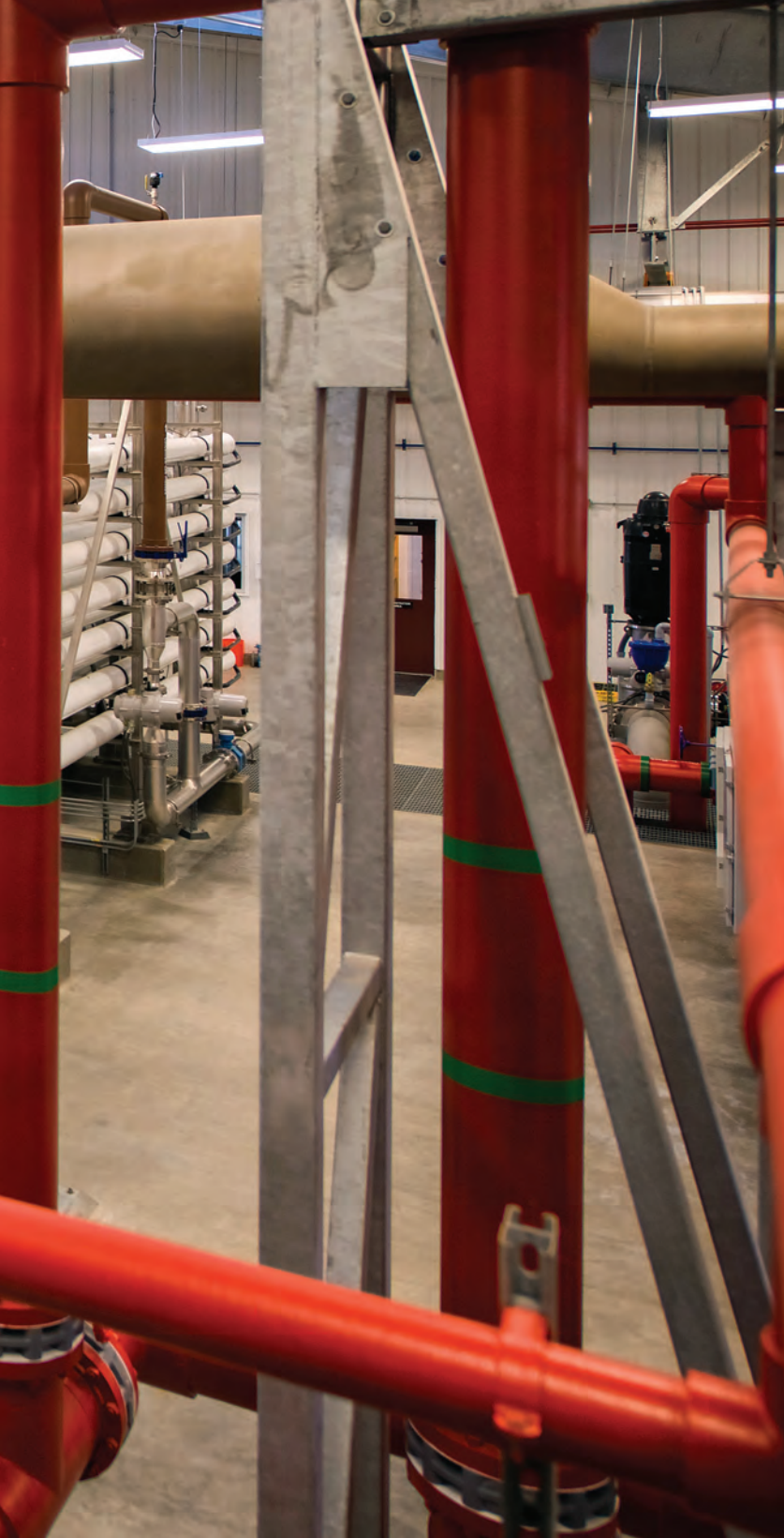
David Beck, left, lead operator, and Jeff Reeves, utilities superintendent, with the reverse osmosis membrane filter array, framed by red RO treated water pipes (H2O Innovation).
