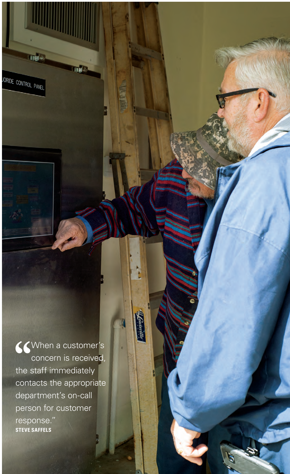
Paul Cockrell, left, maintenance foreman, and Patrick Murphy, chief plant operator, discuss fluoride PLC settings on a C-more touch-screen panel (AutomationDirect).
