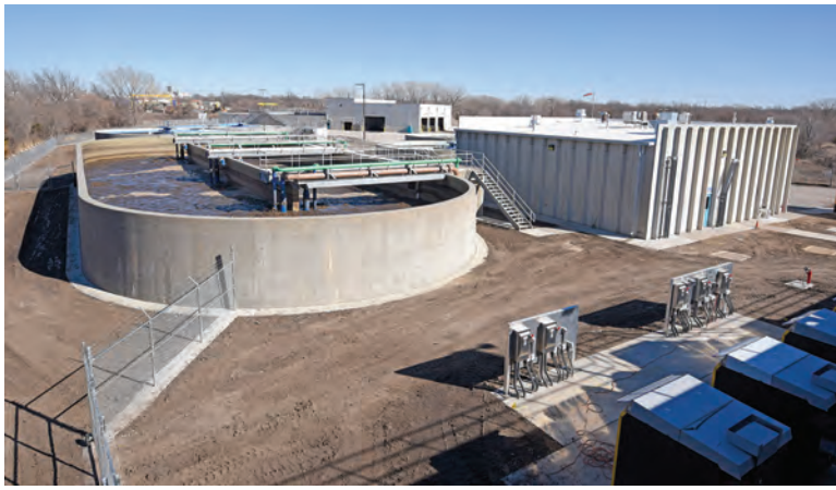
An aeration basin at the Newton treatment facility.
