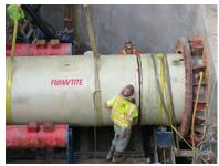
method. This gives outstanding strength and allows for a range of pressure and stiffness classes, as well as different dimensions and lengths. It comes with easy-to-assemble couplings with REKA gaskets. The result is a product that boasts a life expectancy of 150 years. It helps save time and money from day one and throughout the life of the product.
