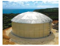
dome covers are all aluminum, maintenance free, corrosion resistant and provide superior field performance.
