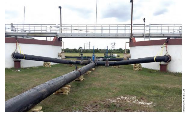
Flow from the aeration basins transfers by way of a 24-inch pipe to 18-inch lines that discharge to the east and west clarifiers at the back of the plant. In the background is the 18-inch crossover pipe that is used to help equalize the clarifiers during elevated flows.
