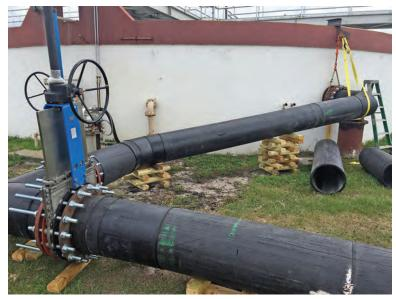
An 18-inch knife gate valve controls the flow from the 24-inch pipe feeding an 18-inch line to a clarifier.
