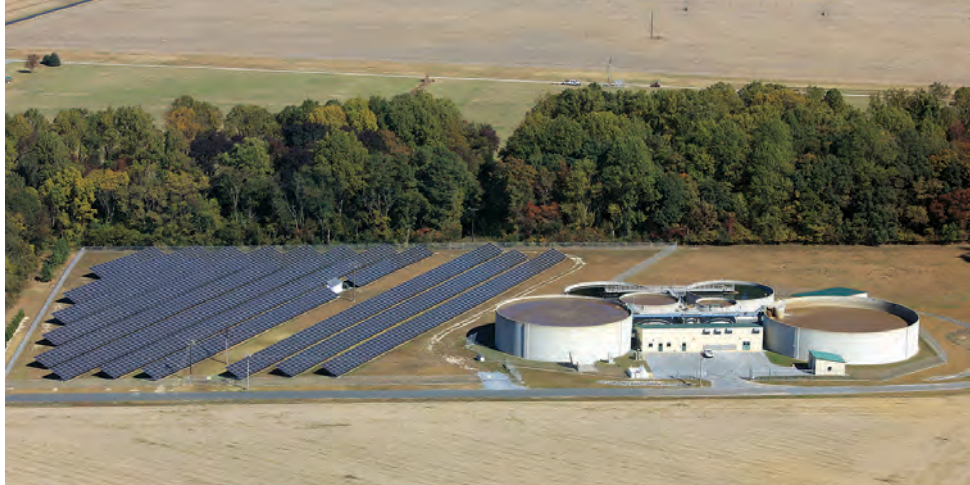
The $2 million solar array at the Hurlock Wastewater Treatment Plant will provide 1.4 million kWh a year and save the plant about $500,000 over 20 years.
