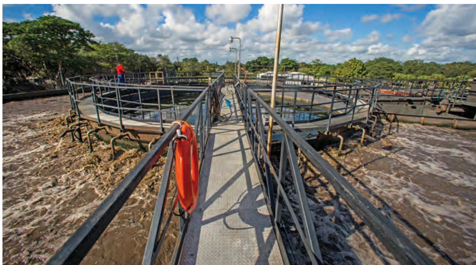
The Hollywood Reservation Wastewater Treatment Plant uses an extended aeration process. It is about to undergo an expansion to accommodate growth.
