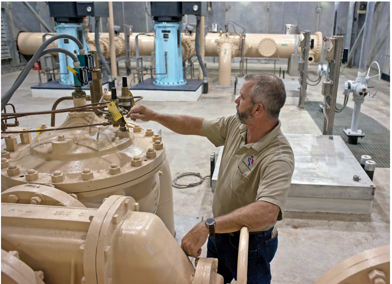
Donald Malovets at the intake area building next to Granger Lake.
