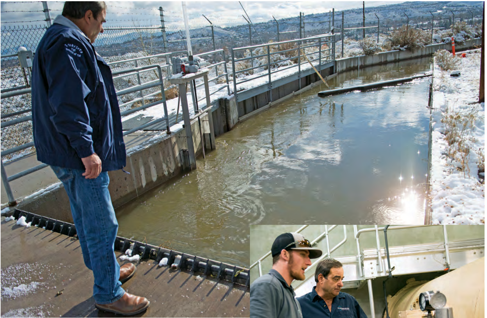
ABOVE: Scott Knecht checks bar screens where raw water is delivered. RIGHT: Knecht discusses the rapid mixer and jet diffuser with Dillon Hansen, apprentice operator.
