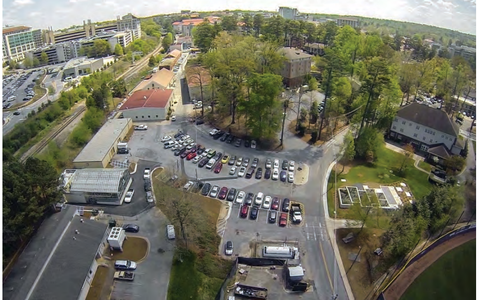
The WaterHub greenhouse (center left) and outdoor treatment facilities (center right) on the Emory University campus reduce potable water use by about 35 percent.
