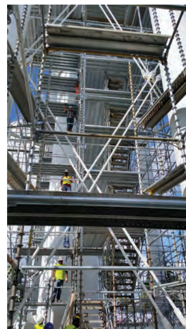
Scaffolding was placed around the tank during the renovation.
