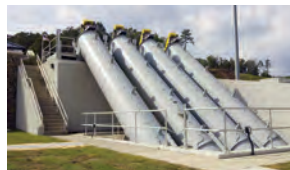
Tube-mounted screw pump from Schreiber
