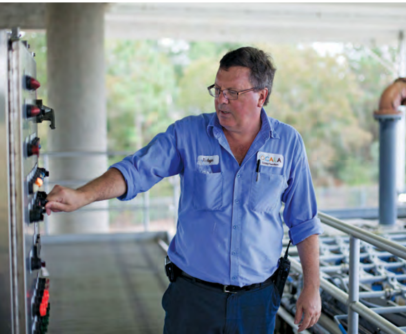
Preston works the control panel for a belt filter press (Alfa Laval Ashbrook Simon-Hartley).
