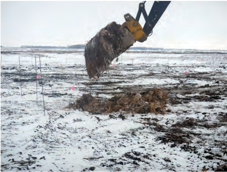
Winter excavation during the early phase of wetland construction.
