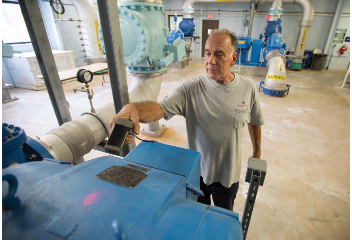
Stephen Koblos, uses an infrared thermometer (OAKTON Instruments) as part of predictive maintenance on a pump motor (Marathon Electric Motors).
