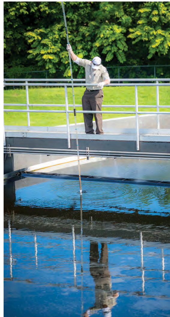
The Eustis plant's step-feed biological nutrient removal process went online in 2012. Tertiary filtration polishes the effluent for distribution through a reuse system that serves golf courses, parks, sports fields and residential landscapes.
