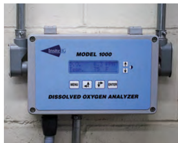
A dissolved oxygen meter continuously monitors lagoon oxygen levels.
