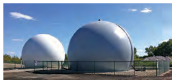
Double Membrane Biogas Holder from JDV Equipment Corporation
