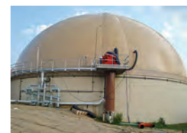
DuoSphere Dual Membrane Gasholder from WesTech Engineering
