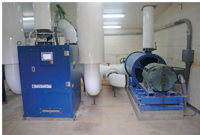
One of the city's new 150 hp Aerzen turbo blowers (left) next to an older 200 hp centrifugal blower installed in 1994.
