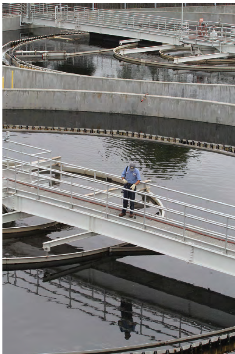
Operator John Bontrager checks the sludge blanket in one of the facility's secondary clarifiers.
