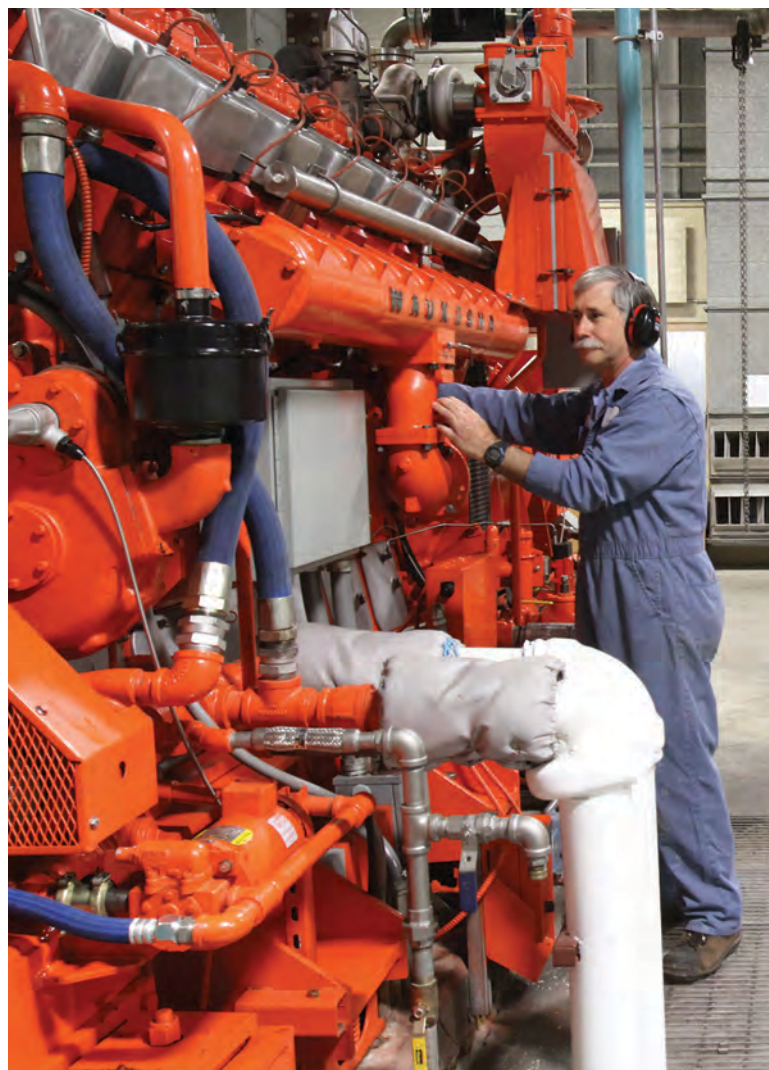
ABOVE: Al Locatelli, mechanic technician, services a Waukesha engine (GE Energy) in the plant's cogeneration facility. BELOW: Michelle Courtroul, lab technician, weighs filters to measure TSS.
