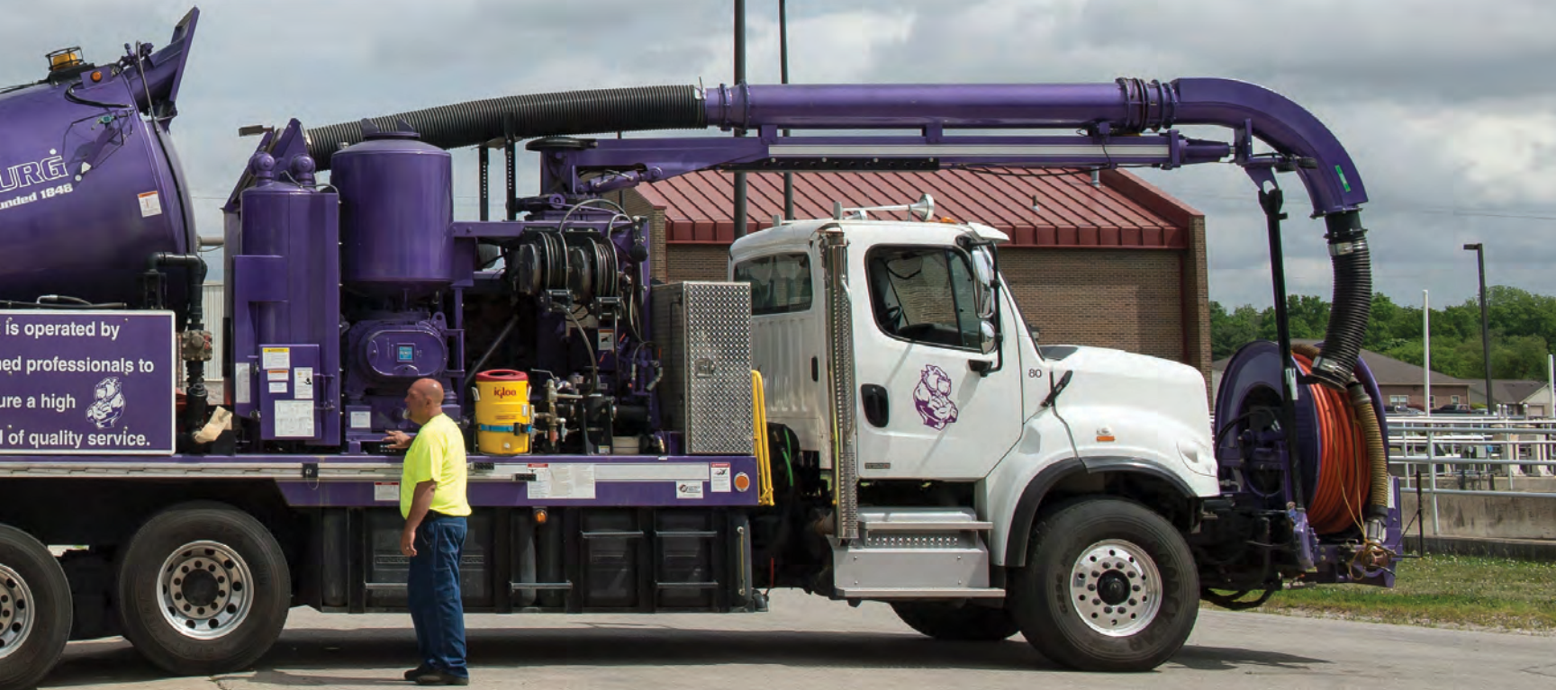
Bill Shaw Jr. (left) and Steve Wyland of the Brownsburg Wastewater Treatment Plant empty the facility’s Vac-Con combination truck after servicing area sewer systems.
