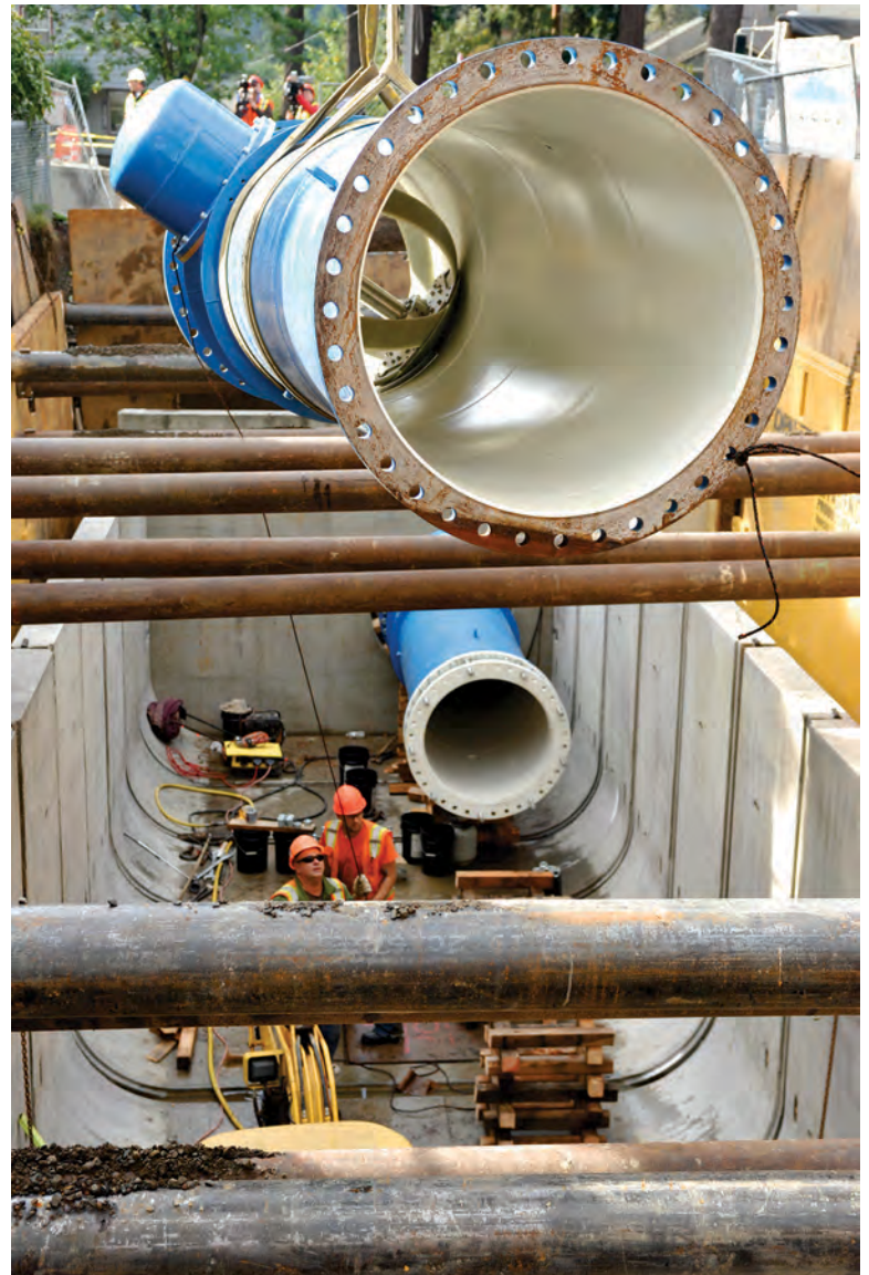
The LucidPipe electrical generating systems were part of a Portland Water Bureau $150 million upgrade. Lucid Energy financed the installation and sells the electricity to the local utility, Portland General Electric
