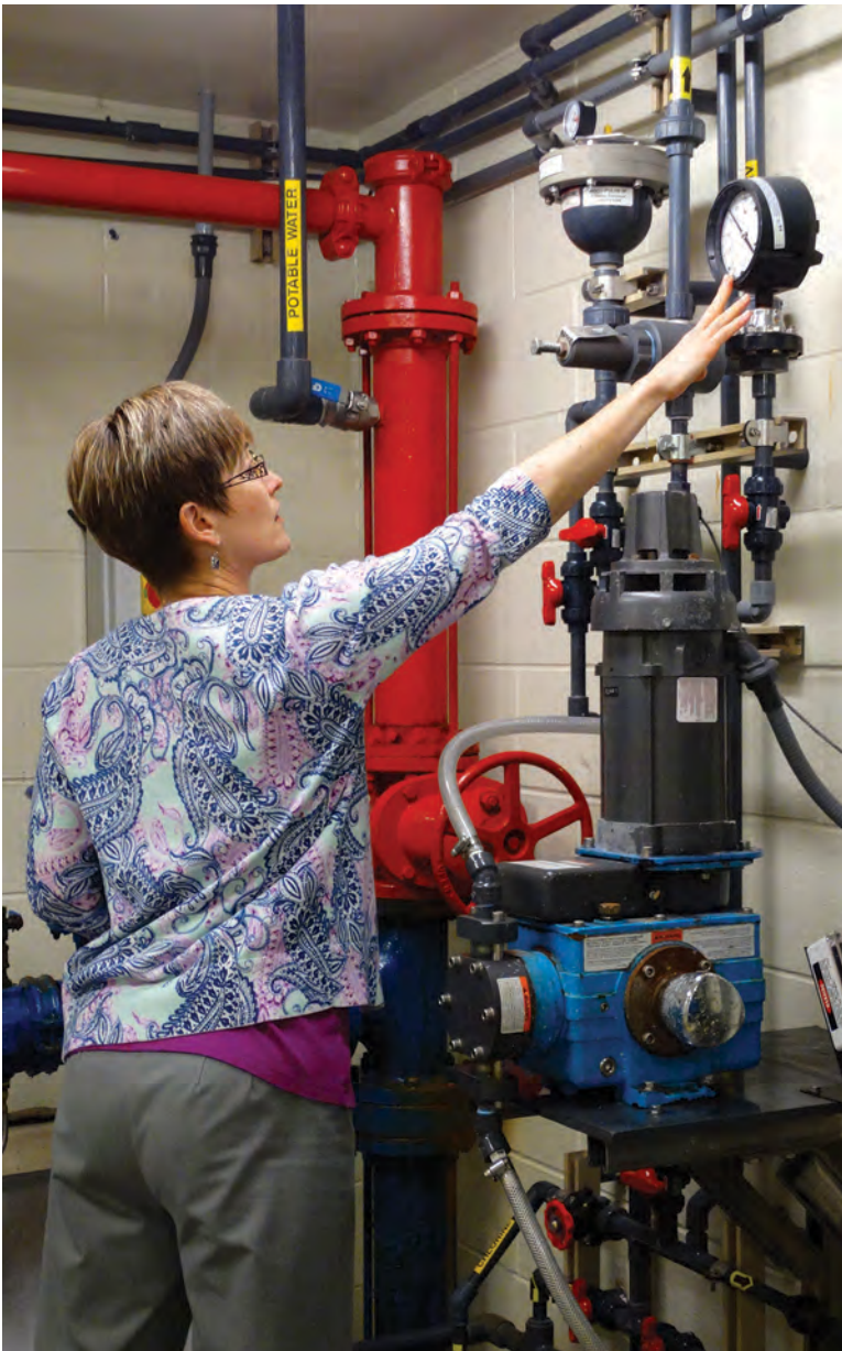
ABOVE: While leading the North Fork team, Carreiro has found time to serve the North Carolina Waterworks Operators Association as a chair of several committees and as president in 2010-11. LEFT: In the chlorine feed system room, Carreiro monitors the pressure gauge of a chemical pump's discharge line (sodium hypochlorite).
