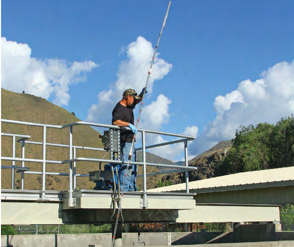
John Pottenger checks the sludge blanket in a final clarifier.
