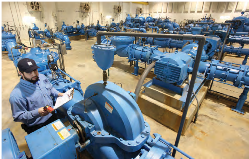
Chris Ashmead checks bearings in the pump room (horizontal split pumps by Pentair - Fairbanks Nijhuis).
