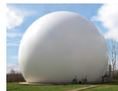
VSO Biogas Technologies gasholders from Geomembrane Technologies
