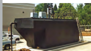
Package wastewater treatment system from Pollution Control Systems
