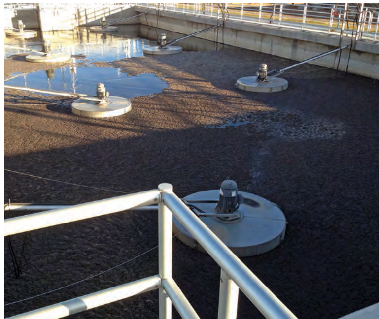
Foam on the surface of the anoxic reactor tank is bulking sludge caused by a booming Microthrix parvicella population.
