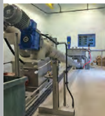
Spiralift SR septage receiving system from Franklin Miller
