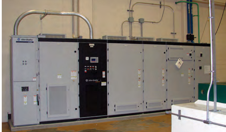
New variable-frequency drives have significantly improved the old blower's efficiency by enabling modulation of blower output.
