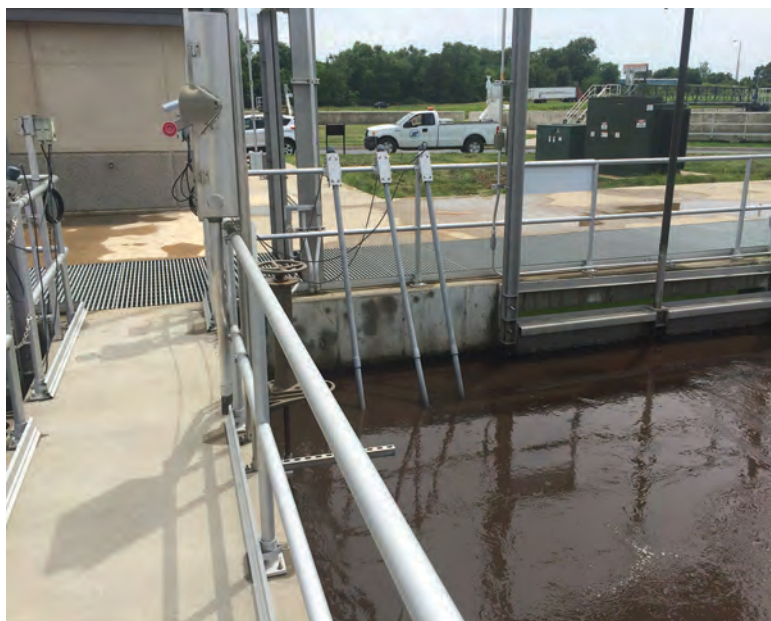
IQ SensorNet probe/arm assemblies monitor dissolved oxygen, pH and oxidation-reduction potential.
