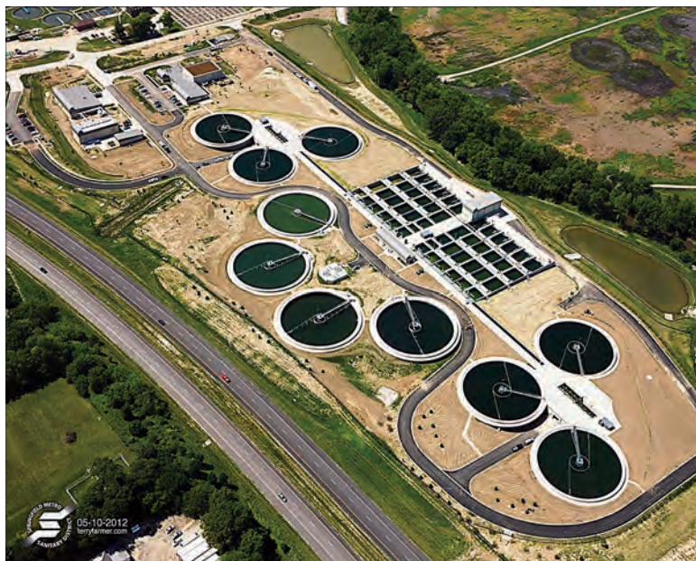
The Spring Creek Wastewater Treatment Plant in Springfield treats 32 mgd with vertical-loop reactor technology.
