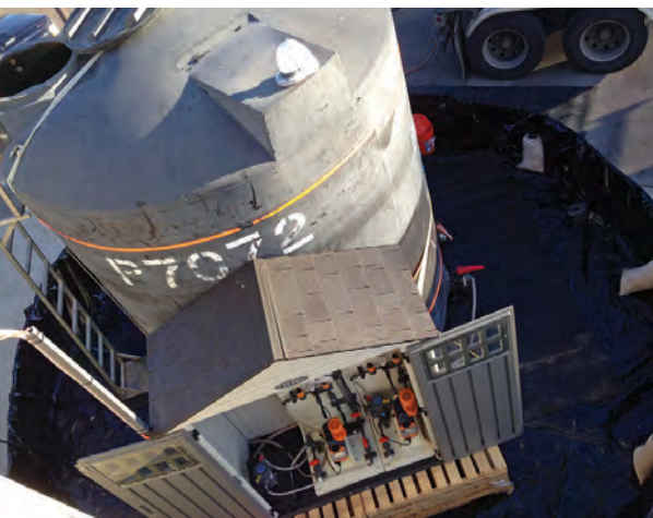
The FEX-208 storage tank and dosing equipment.
