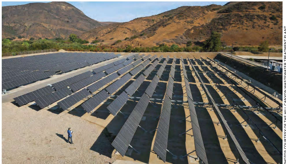
ABOVE: The Hill Canyon Wastewater Treatment Plant’s 2,783 solar panels utilize a motorized system to track the sun as it travels across the sky in order to maximize electrical generation.
