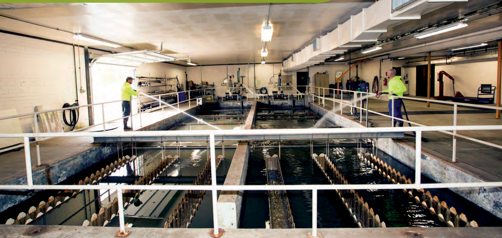
Dennis Jones and Justin Haley clean the final clarifiers.
