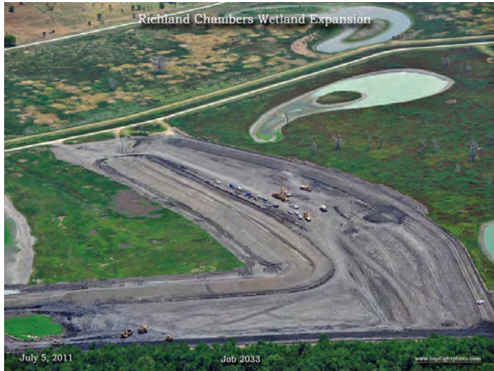
The Richland-Chambers Wetlands under construction (left) and after completion.
