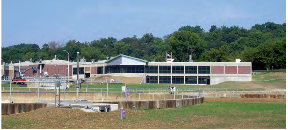
The renovation of the Dubuque Water & Resource Recovery Center included a new administration and laboratory building with a heating and cooling system that uses effluent heat recovery.
