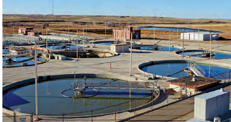
The River Road plant (above) and the Hollywood Road plant both use a conventional activated sludge process.
