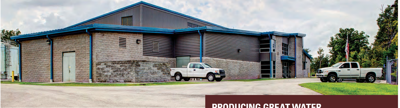
The J. Isom Lail Water Treatment Plant.
