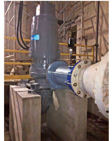
ABOVE: Workers install a new aeration diffuser (Environmental Dynamics International) as part of an update to one of the four PRASA wastewater plants covered by energy performance contracts with Honeywell. RIGHT: New wastewater pumps (Flygt) installed across the PRASA wastewater treatment plants include this 2,000 hp, 100 mgd pump.
