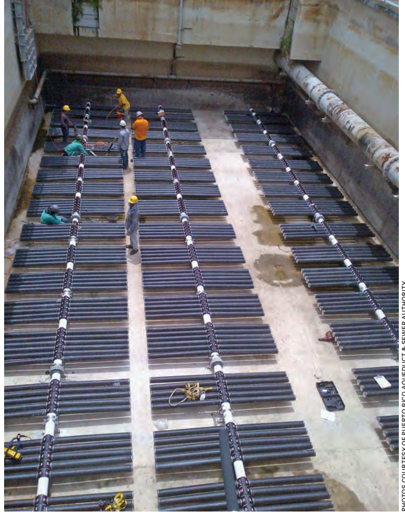
ABOVE: Workers install a new aeration diffuser (Environmental Dynamics International) as part of an update to one of the four PRASA wastewater plants covered by energy performance contracts with Honeywell. RIGHT: New wastewater pumps (Flygt) installed across the PRASA wastewater treatment plants include this 2,000 hp, 100 mgd pump.
