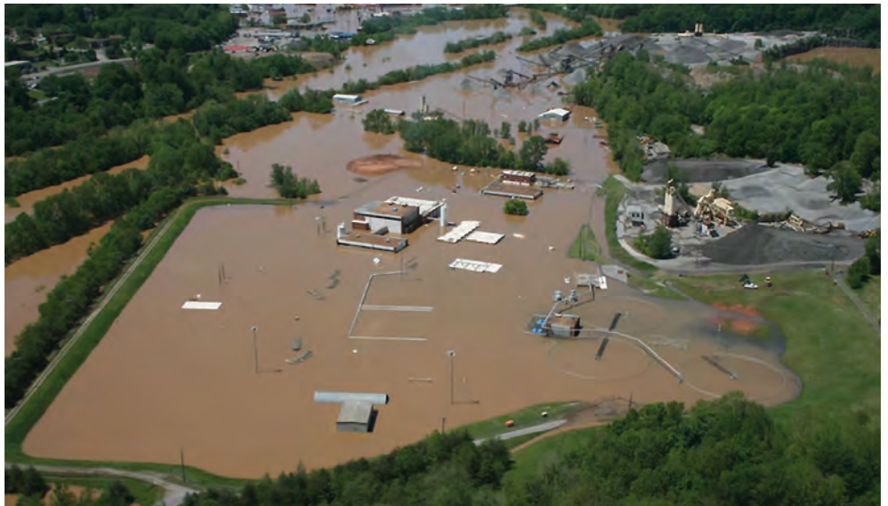
During the May 2010 flood, the Cumberland River over-topped a berm and filled the bowl in which the Clarksville treatment plant lies.
