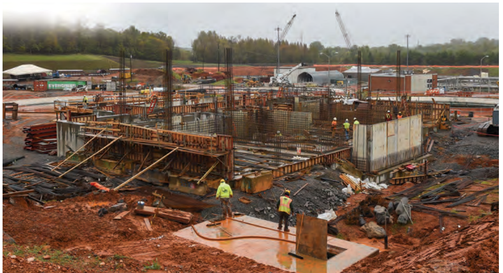
A new headworks building is under construction at the Clarksville plant.
