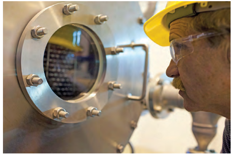
Ozone generators, including this WEDECO Model PDO-3000Y, contribute to the plant's disinfection process.
