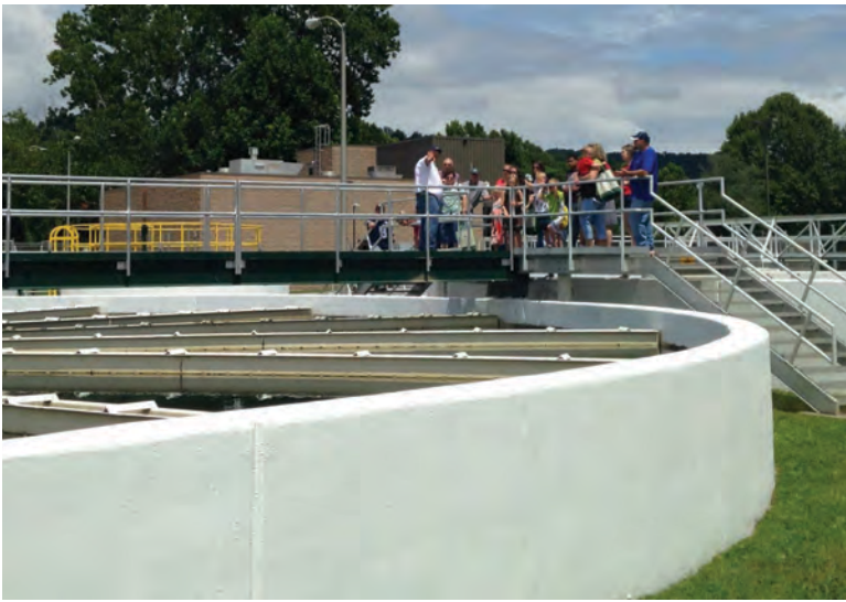
A tour group examines a clarifier at the Kanawha Valley Water Treatment Plant.
