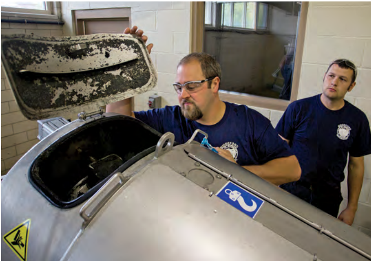
Jon Koestner (left) and Steve Demers check the cake consistency in the Huber screw press during normal maintenance rounds.
