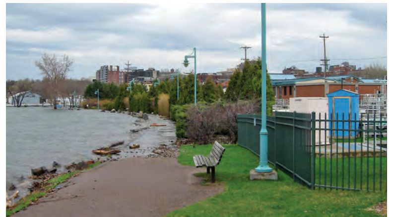
Floodwaters neared the chlorine tank and clarifiers in May 2011.
