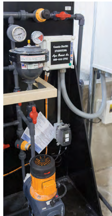
A metering pump (ProMinent) measures chemical dosing for treating water provided to municipalities in St. Clair County, one of the fastest growing counties in Alabama.
