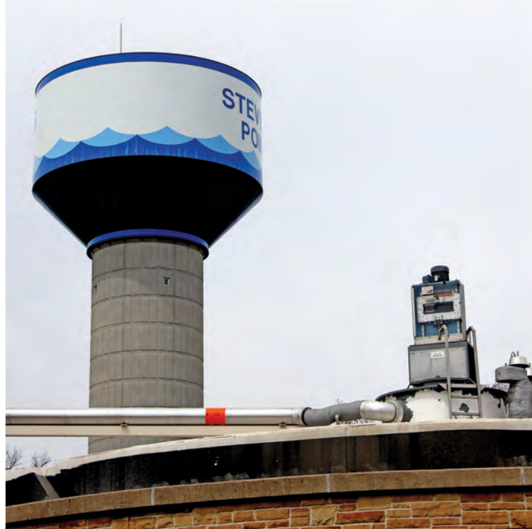
A linear motion mixer (Ovivo) sits on top of digester No. 3 at the Stevens Point Wastewater Treatment Plant.
