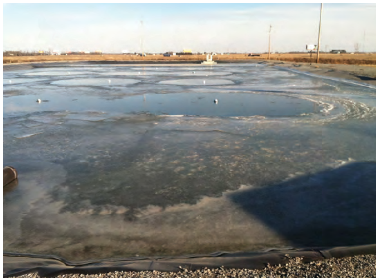
The new lagoon system has functioned well in warm and cold conditions and has reduced ammonia, BOD and TSS to below permit limits.
