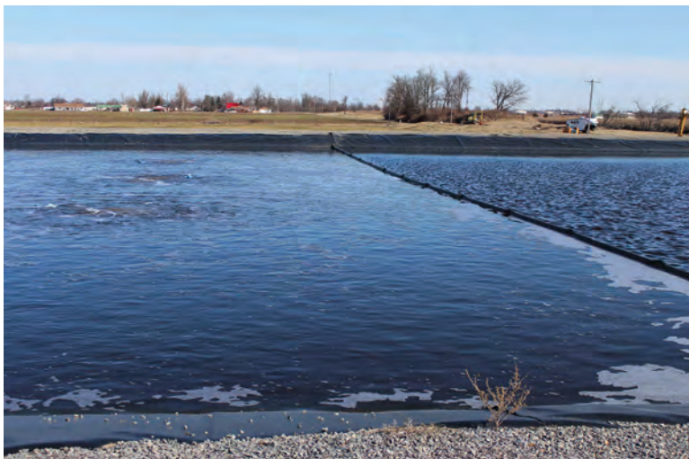
Partial mix zone (left) for sludge management and quiescent zone (right) for solids separation.
