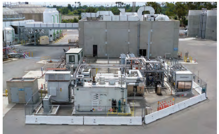
The $8 million tri-generation pilot research project is the first to use digester gas to produce electricity, hydrogen for auto fuel, and heat for anaerobic digesters. It can produce 250 kW of electricity and 100 kilograms of hydrogen per day (equivalent to about 250 gallons of gasoline).
