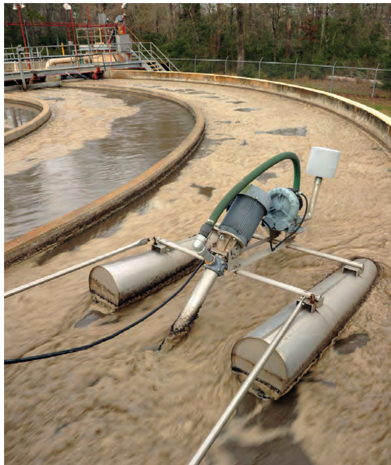
A mechanical aerator keeps solids in suspension and introduces oxygen (Tornado aerators from AEROMIX Systems).
