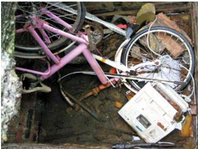
ABOVE: A live goldfish found in a Scottish Water wastewater treatment line. BELOW: A bicycle and a fax machine blocked a sewer drain in East Kilbride.
