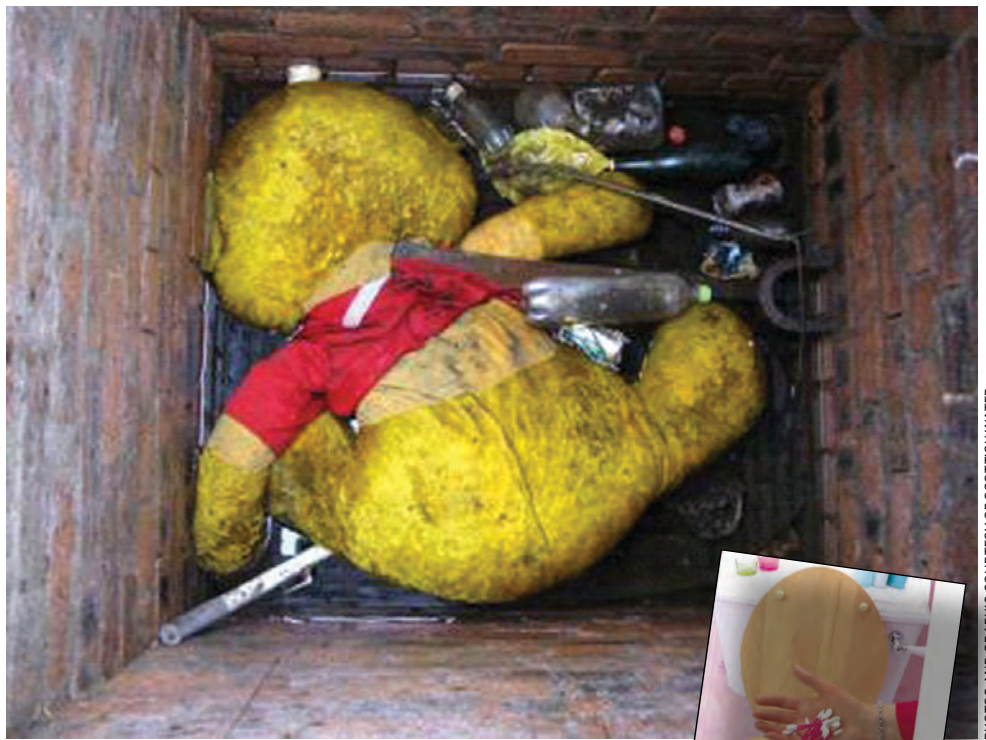
ABOVE: A stuffed Winnie the Pooh backed up a sewer drain in East Kilbride. RIGHT: A Scottish Water educational brochure.
