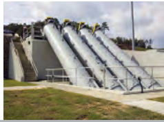
Archimedian Tube-Mounted Screw Pump (TMSP) from Schreiber
